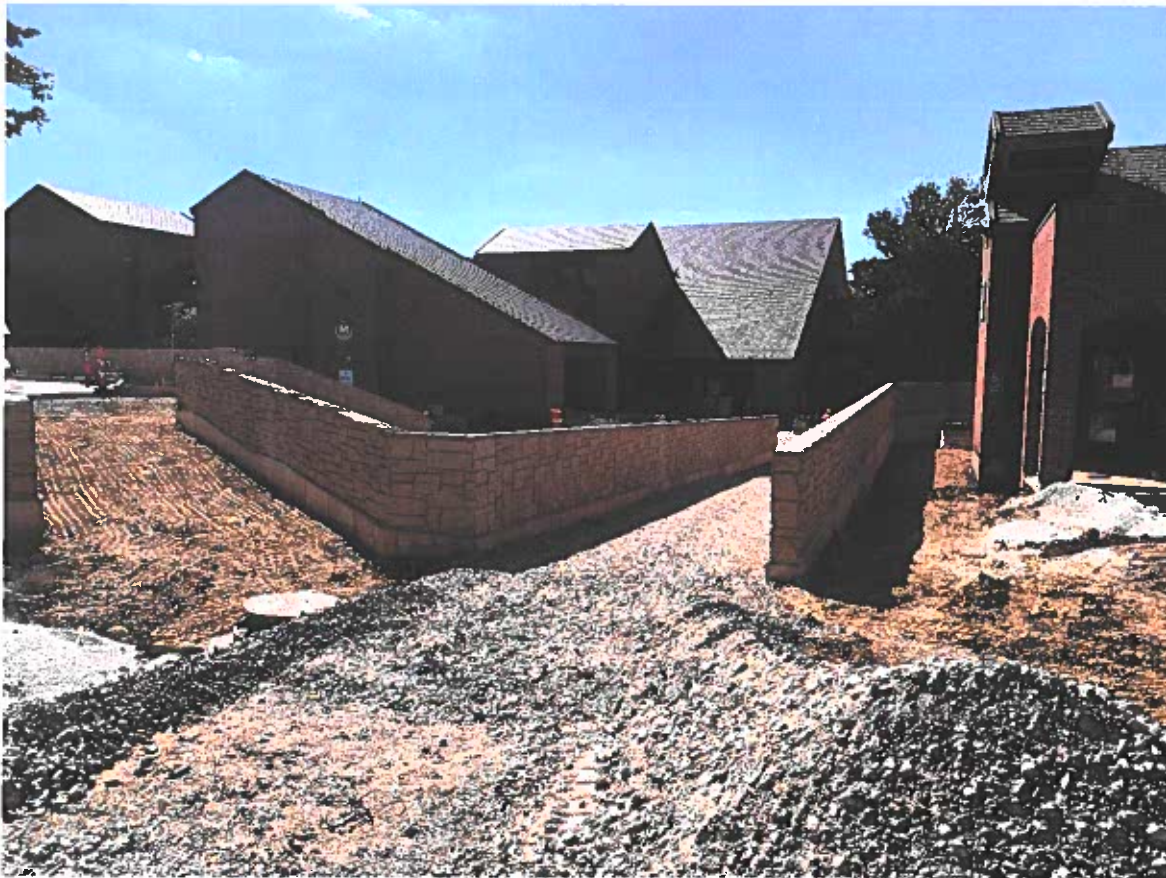
ADA walkways and concrete walls, looking West towards the M Wing
