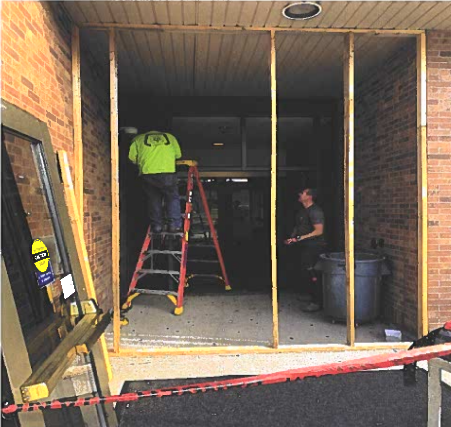
D2 Door replacement in progress
