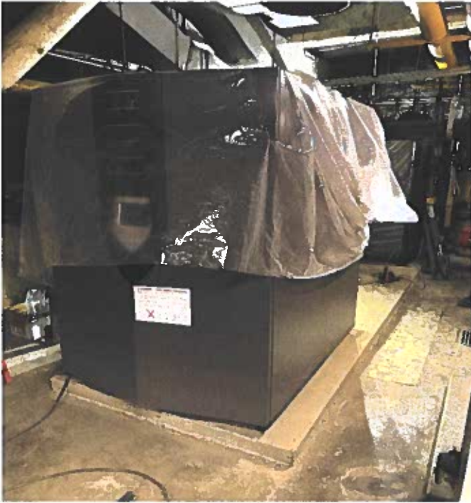
New boiler installation
