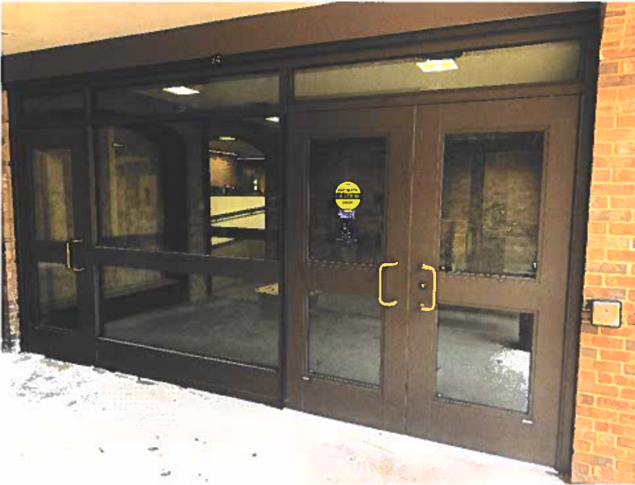
X4 Door replacement completed
