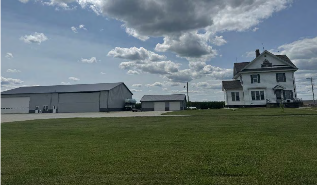
From adjacent property looking west toward subject property (527).
