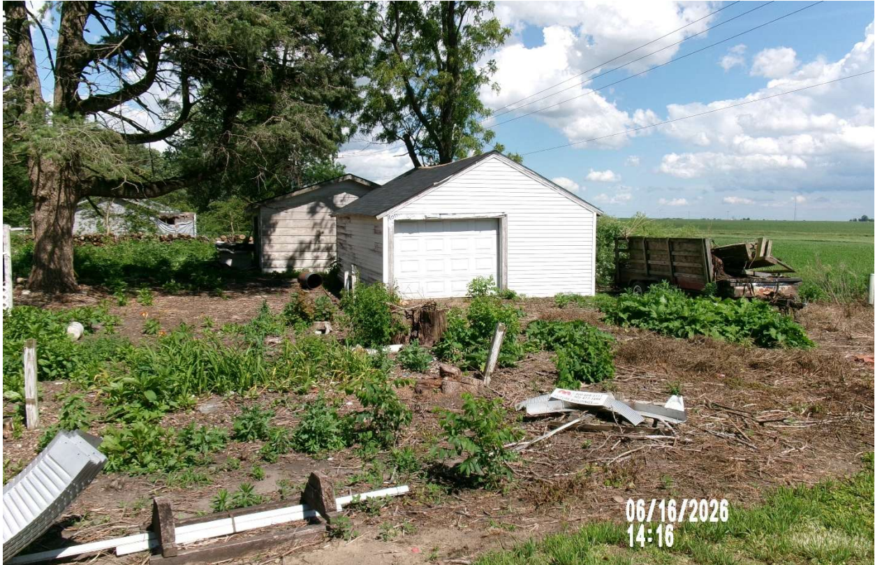
From Third St looking east toward garages on the subject property.
