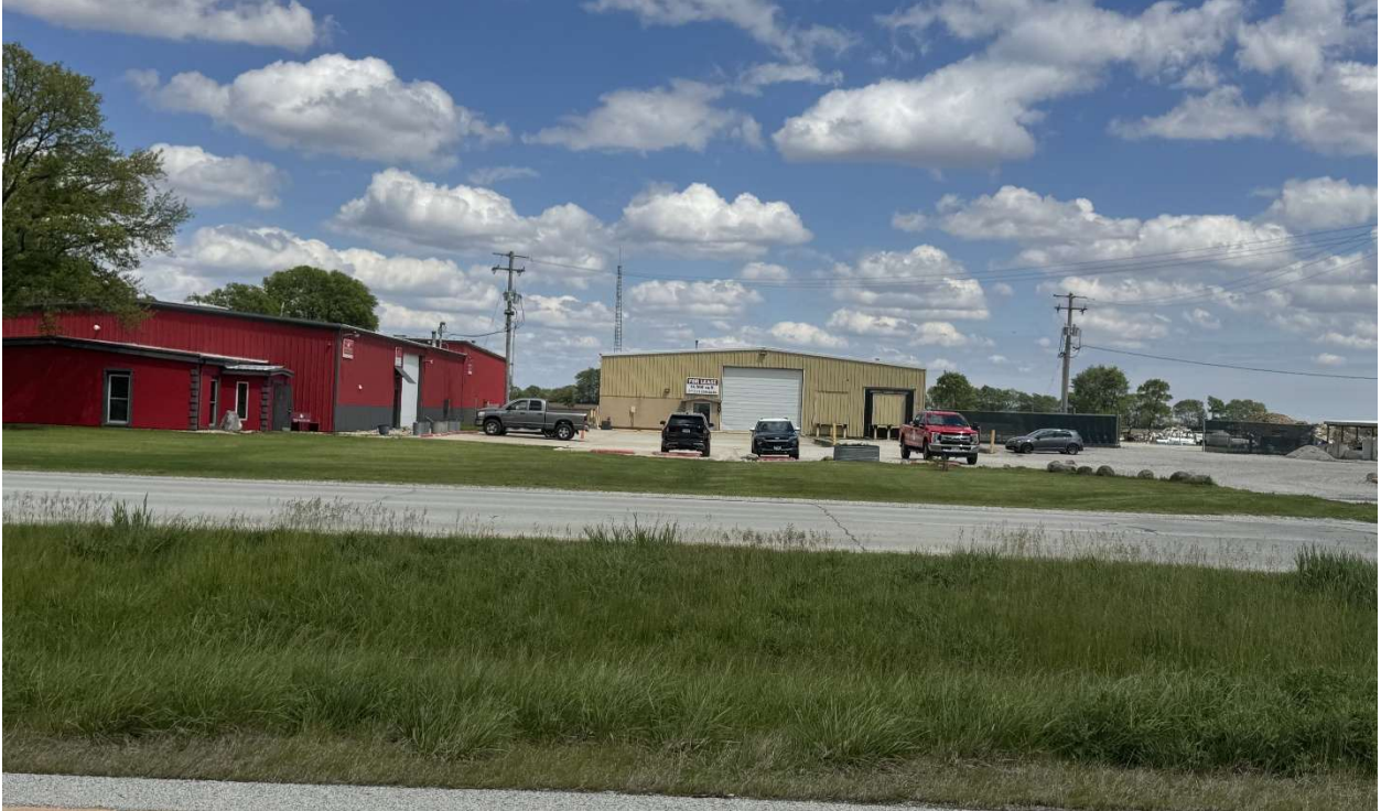
From US-45/N. Cunningham Ave looking east toward 4812 & 4808 N. Cunningham
