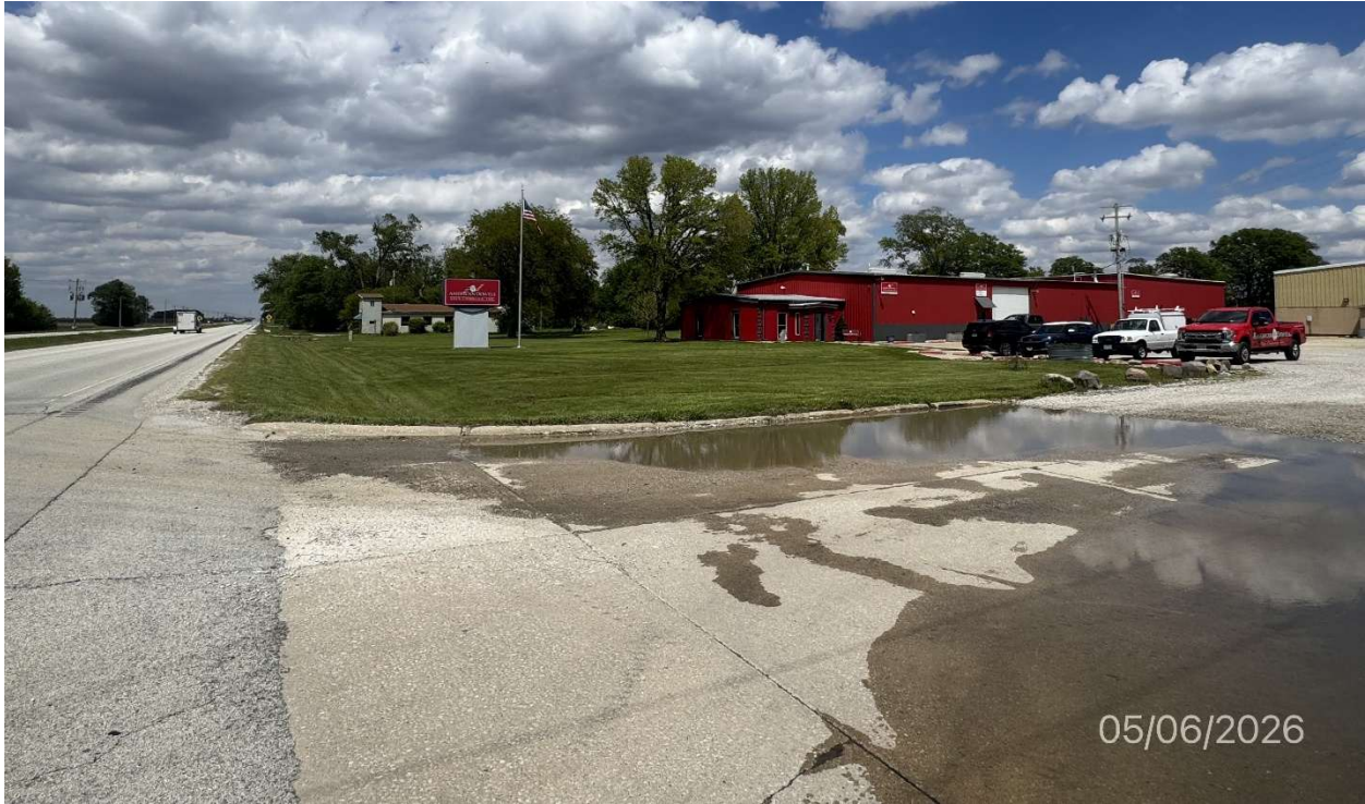
From entrance driveway looking north along US-45/N. Cunningham
