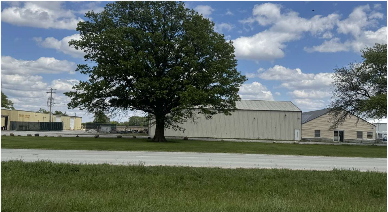
From US-45/N. Cunningham Ave looking east toward 4712 N. Cunningham
