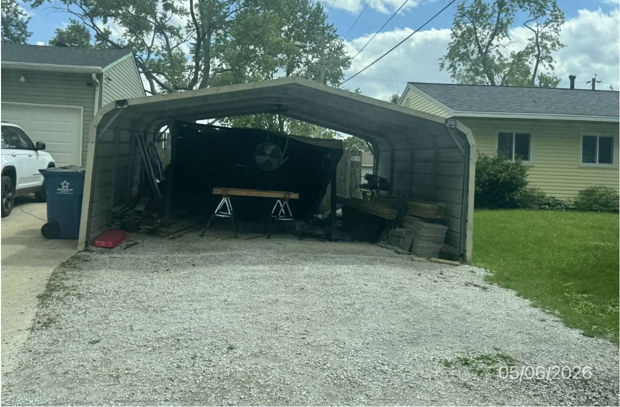
From E Nevada St looking toward carport
