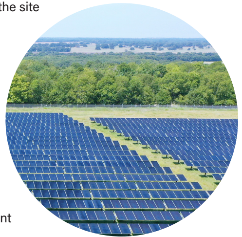
Image provided courtesy of Pattern Energy Group LP
