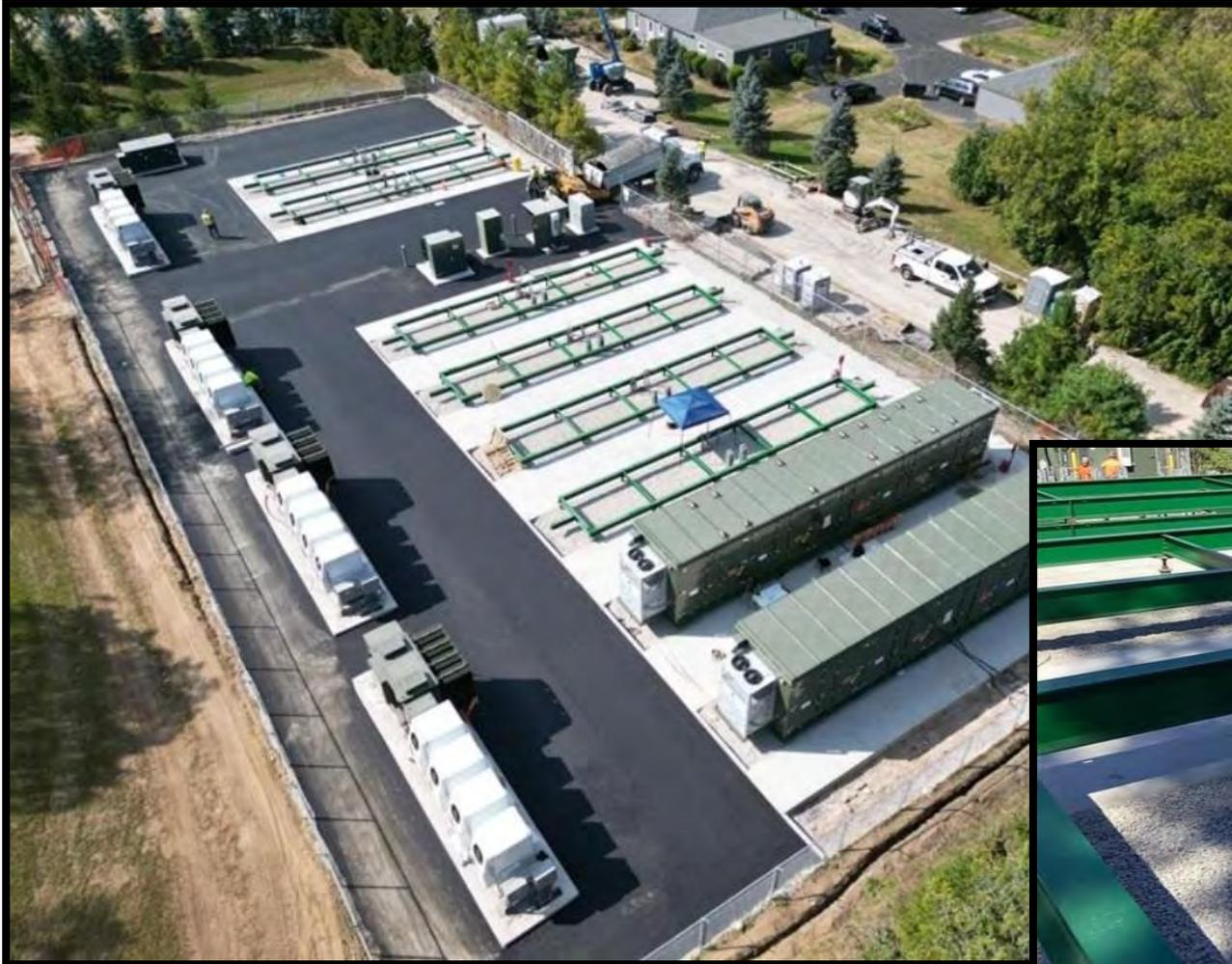
Containers are placed on concrete pads--or increasingly, on steel skid and helical piles
