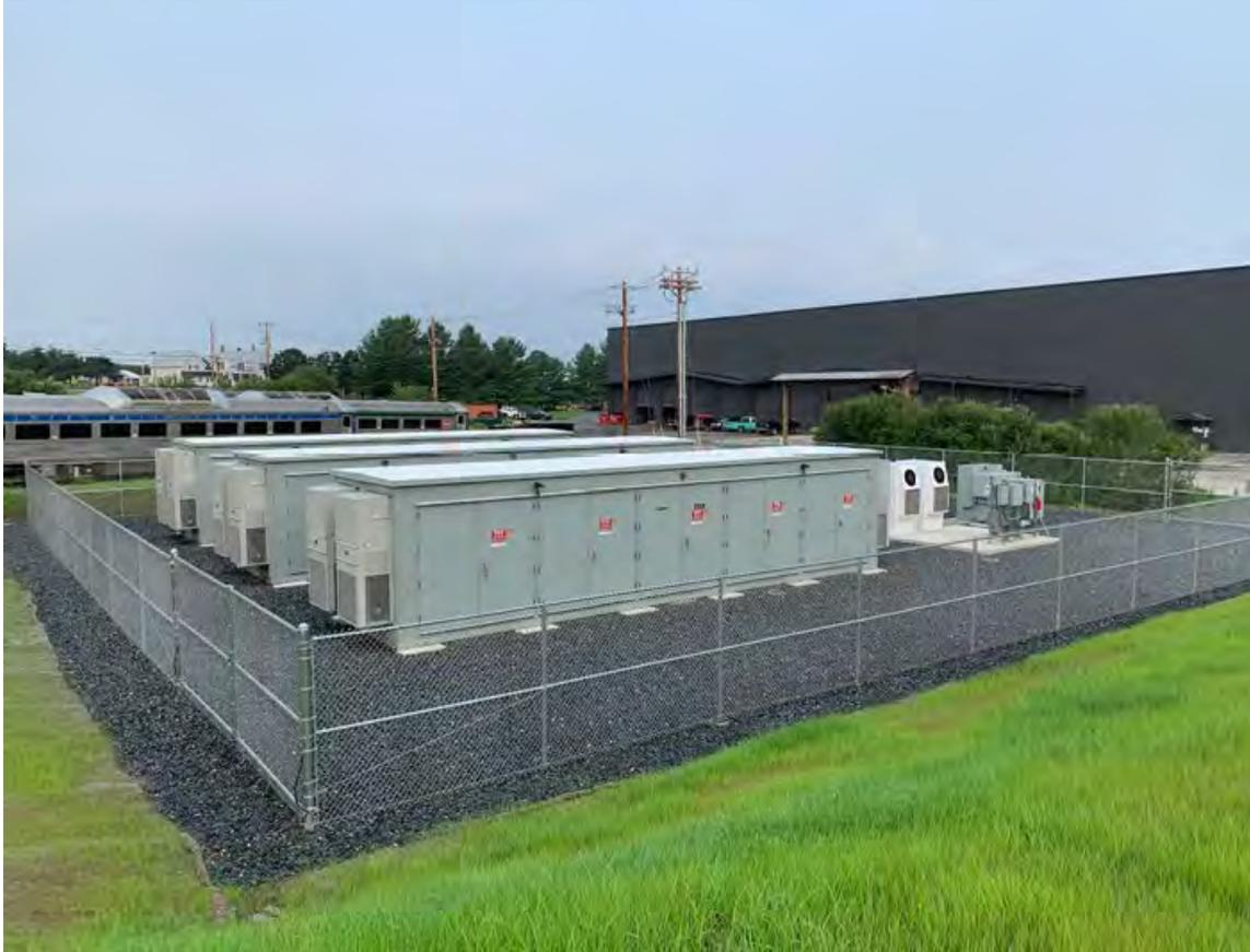
*This utility-scale ESS in Vermont is using li-ion batteries to provide peak reduction and frequency regulation services. Photo courtesy of WEG. Source: Energy Storage Systems based on the IBC, IFC, IRC, and NEC, International Code Council, January 2022*
