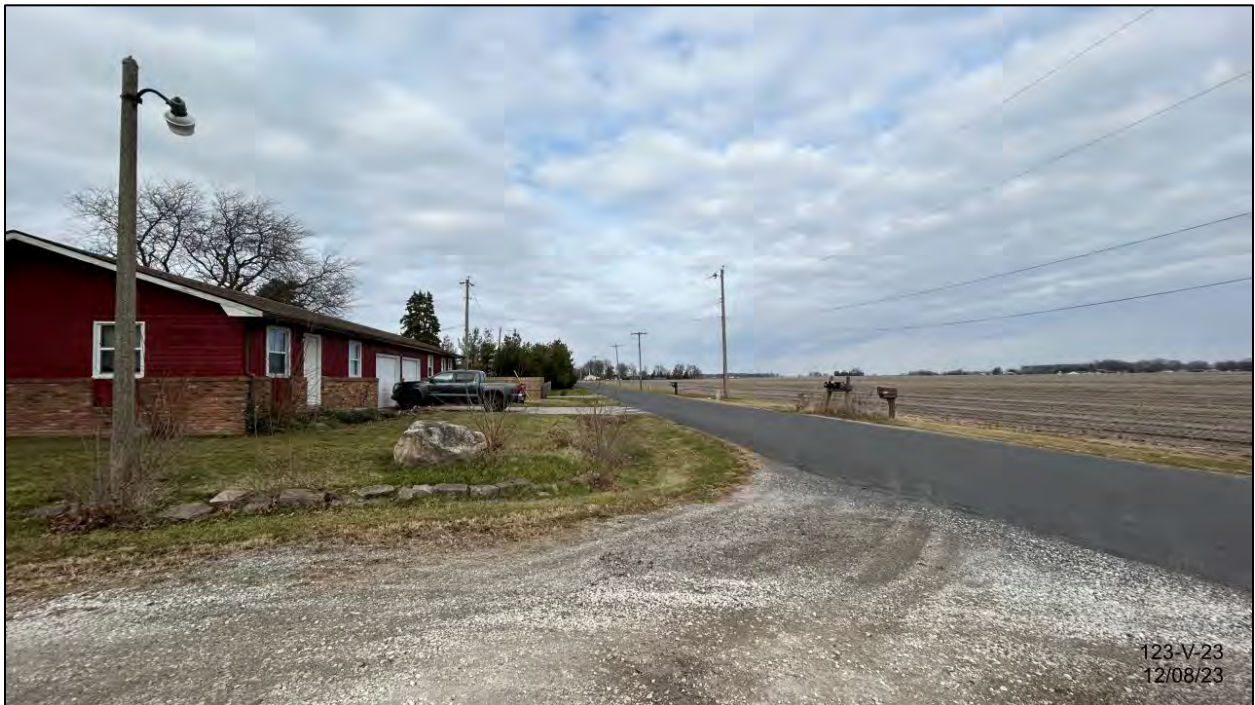
From west of Willow Rd facing north to duplex
