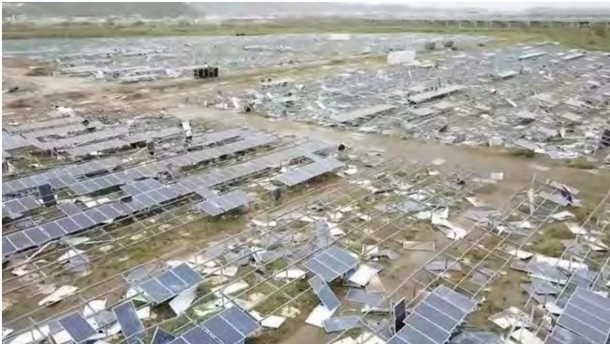
Destroys Solar Farm in Puerto Rico Bob Meinetz
