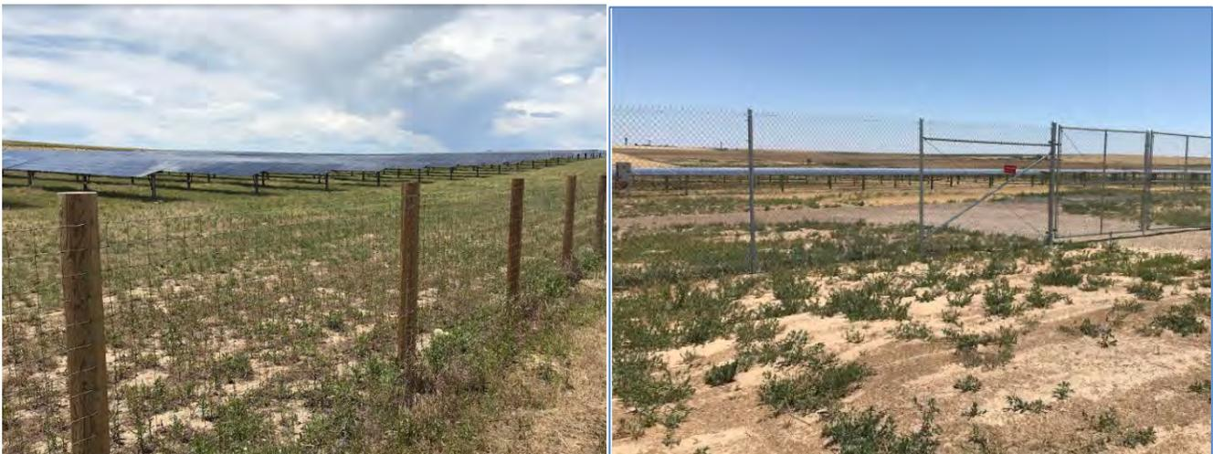
**Photo 2.** Fencing Options including agricultural style fencing (left) or chain link (right).
