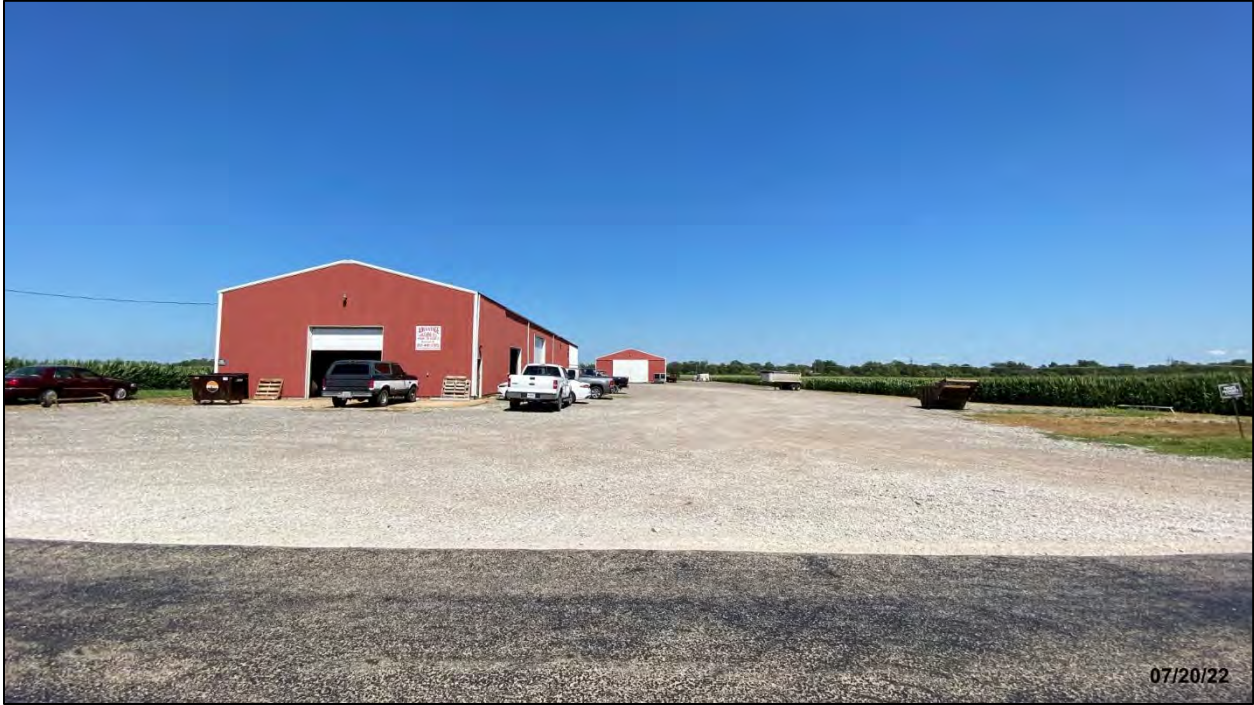
From CR 1500E facing east to subject property
