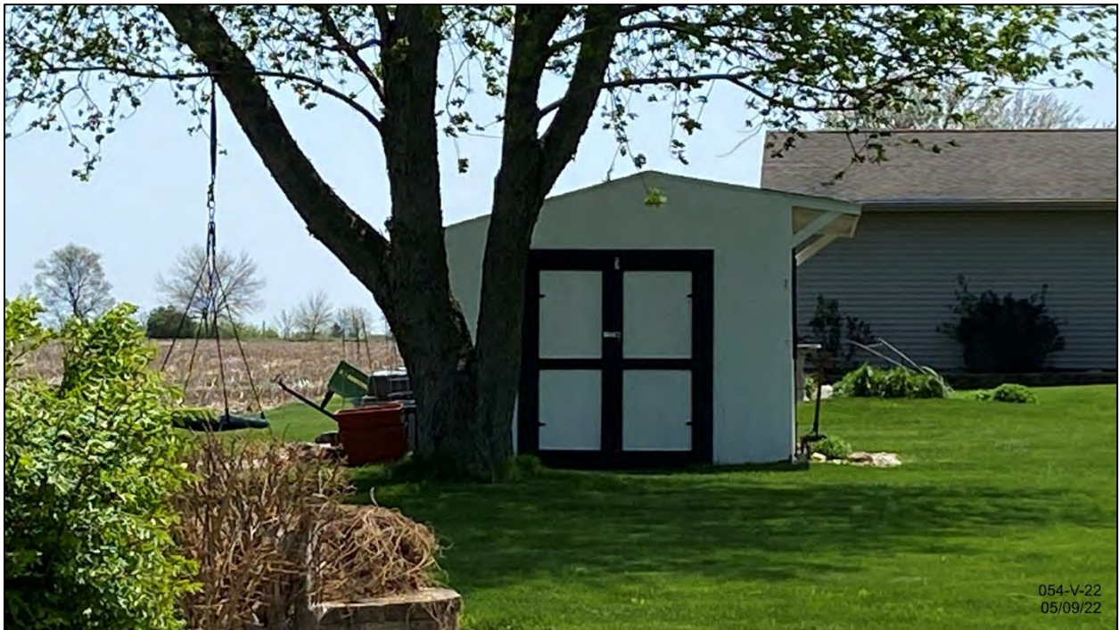
From N Trailside Drive facing south to shed
