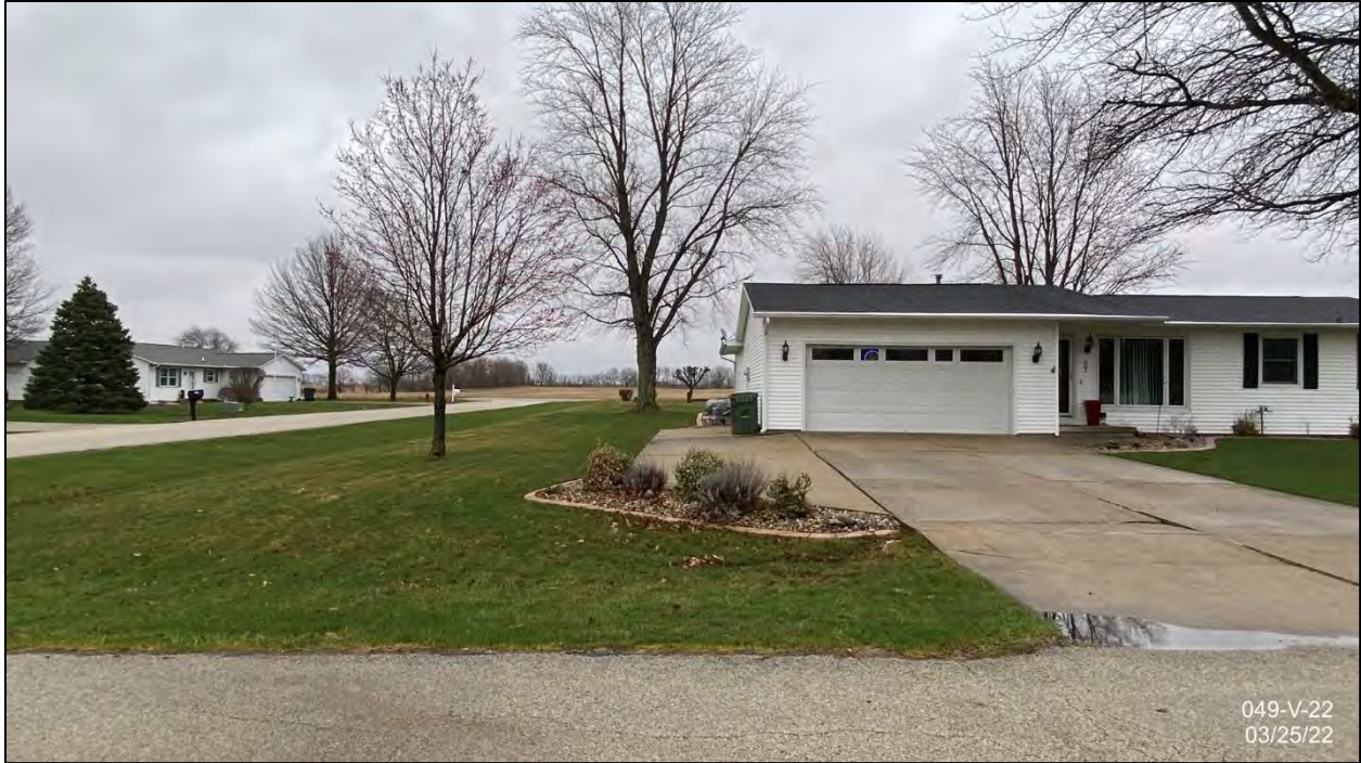
From Surrey Ct facing East to subject property – proposed garage would be left of existing garage
