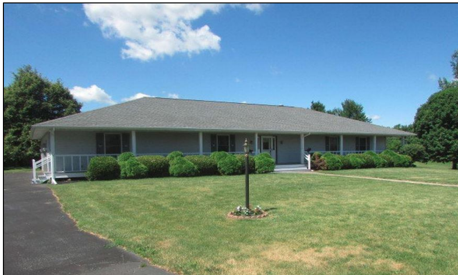
Figure 8: View of residence looking southwesterly from edge of driveway.
