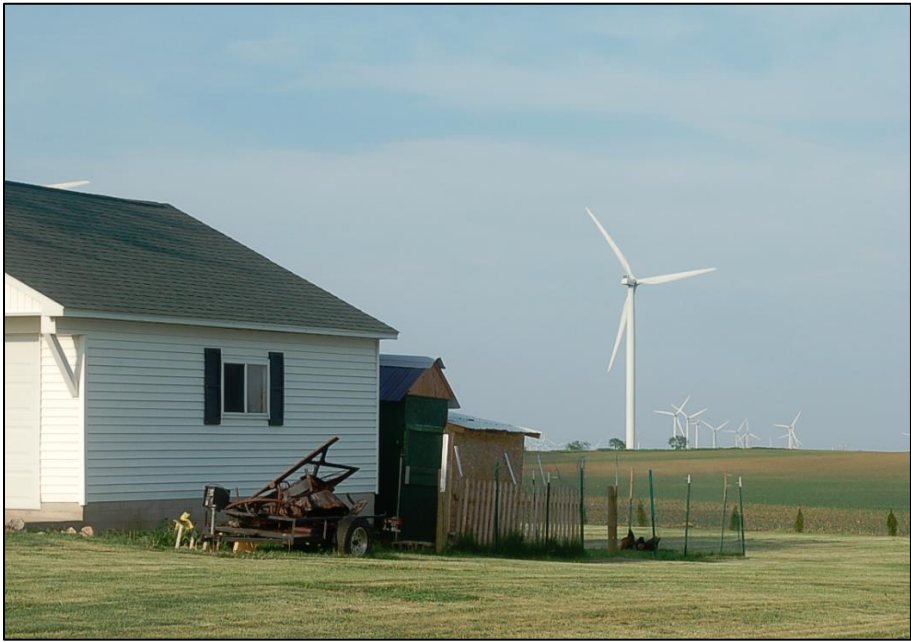
Figure 12: View of Wind Turbines looking northeasterly from southern end of property.
