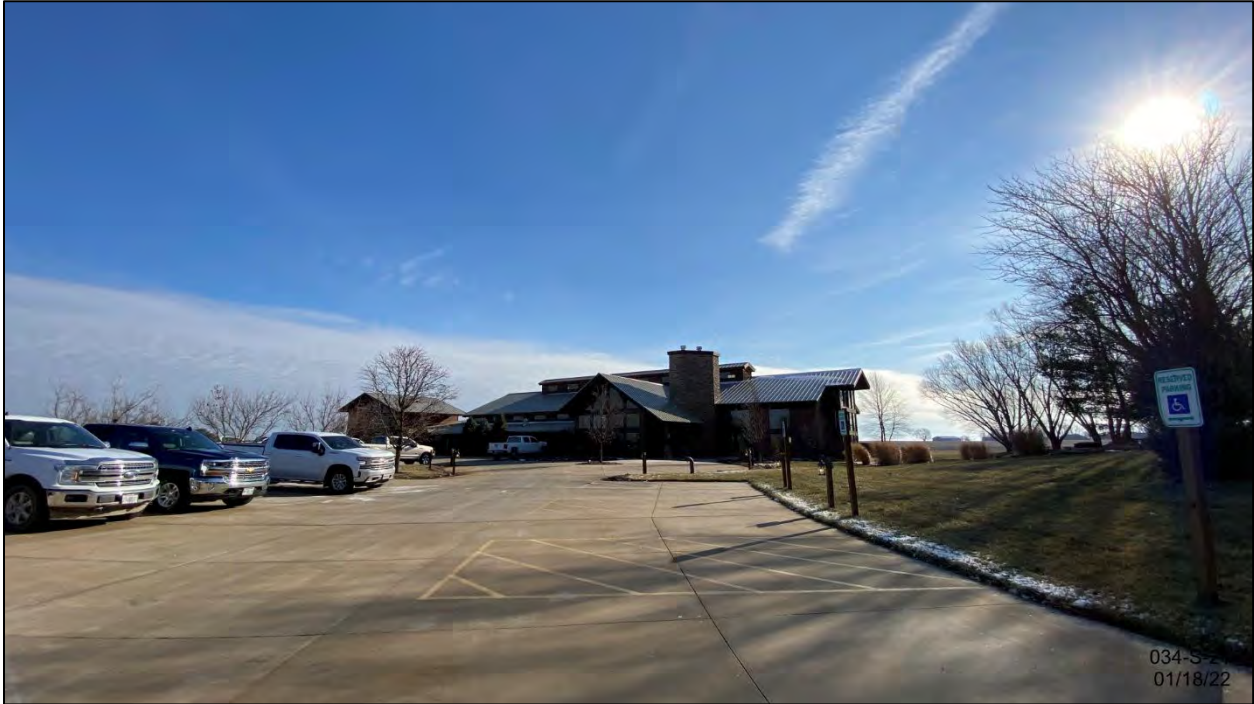
Main event center building at east end of subject property
