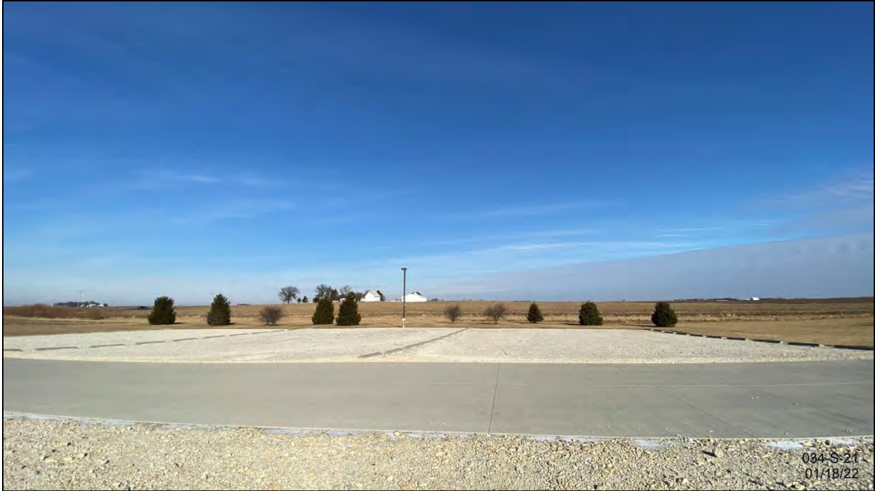
From proposed chapel location facing north showing parking lot screening
