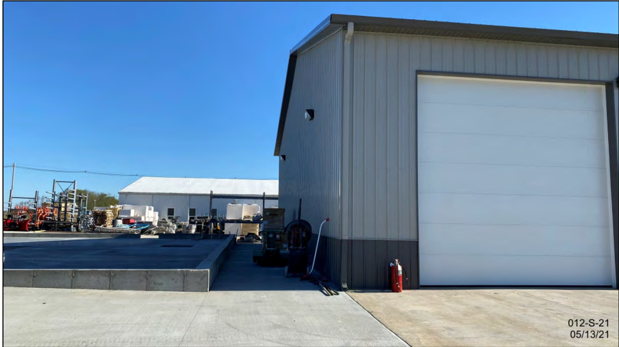
Proposed building foundation to left of newest existing building
