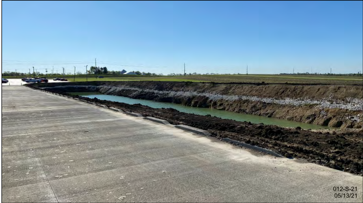
Storm water detention basin south of newest building and proposed building
