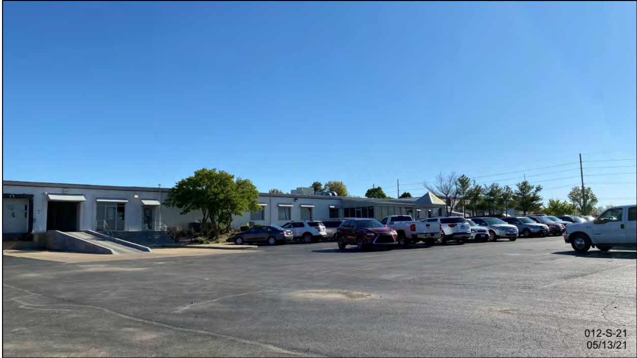
Middle building addition to easternmost building
