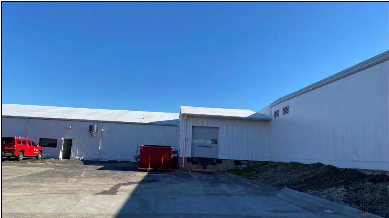
Receiving dock connecting middle addition and original westernmost building
