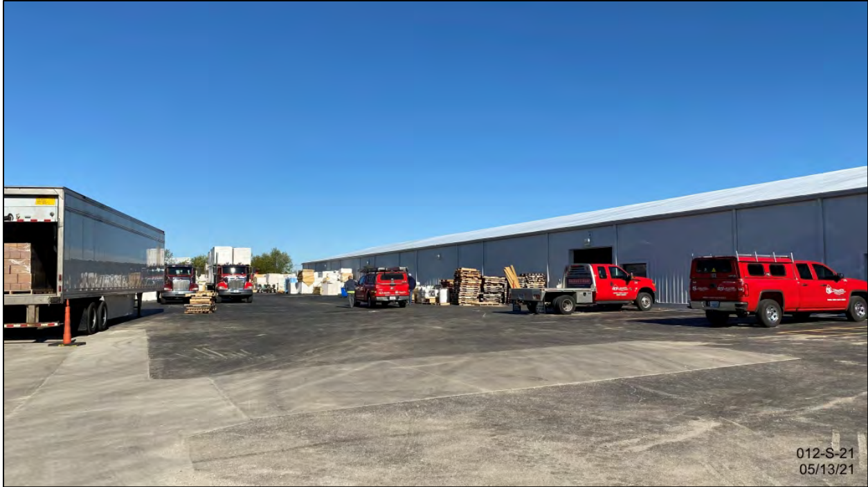
Westernmost original building on north side of subject property
