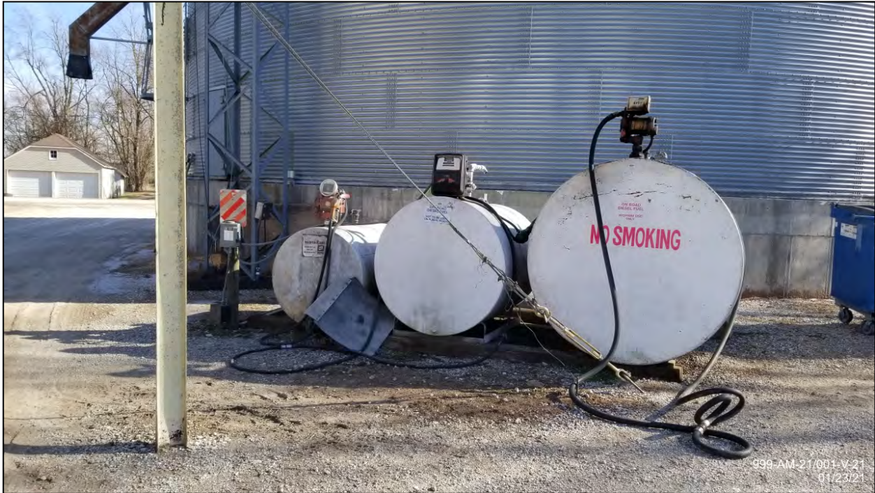
Fuel tanks west of central grain bin
