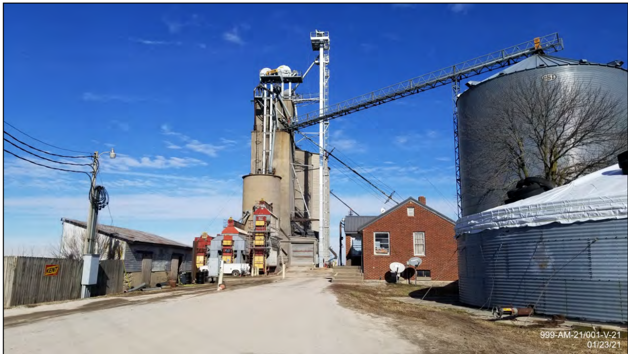
From CR 3050N facing north
