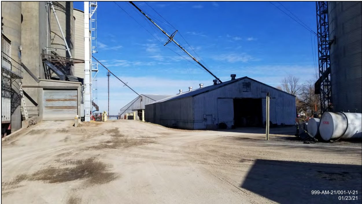
Non-conforming storage building toward center of property
