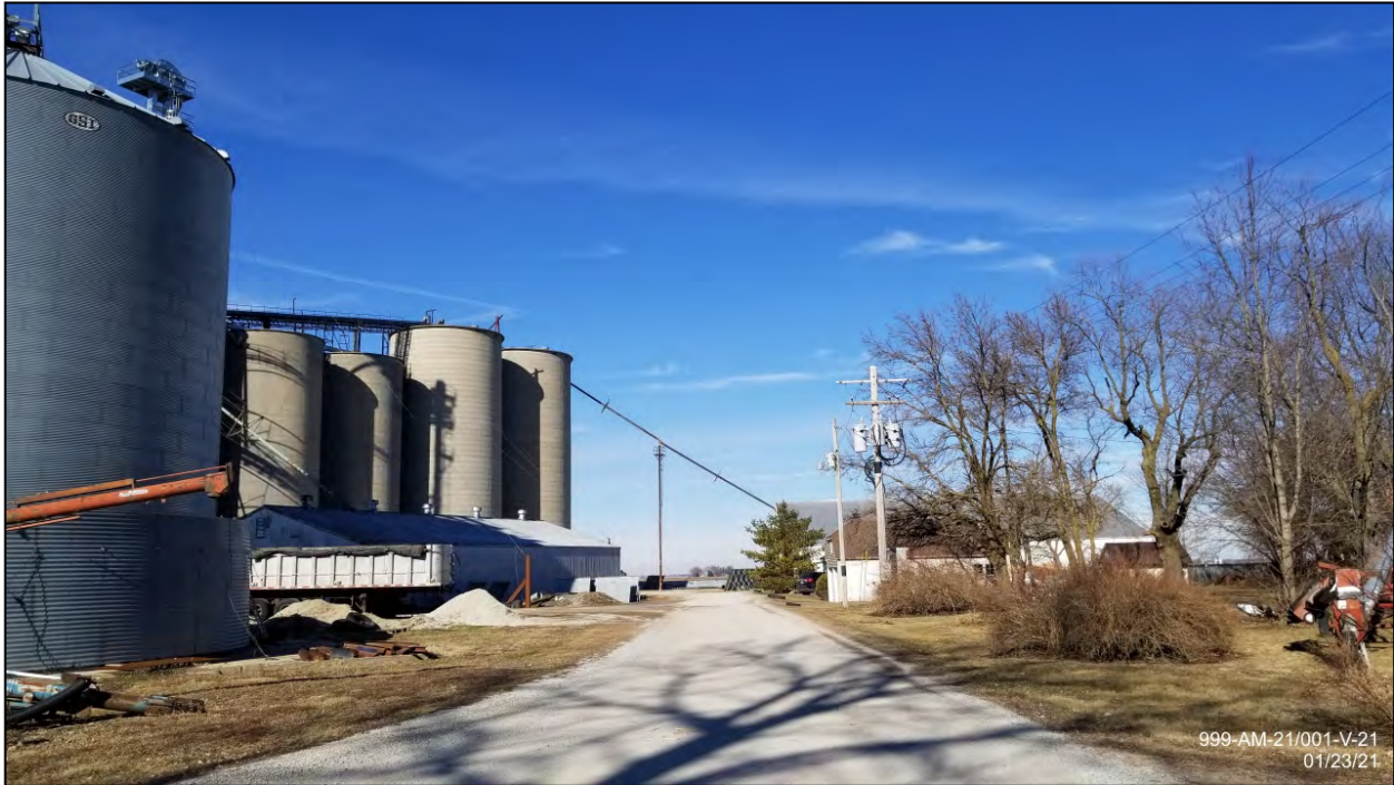
From corner of CR 3050N at CR 3055N (north-south segment), facing north
