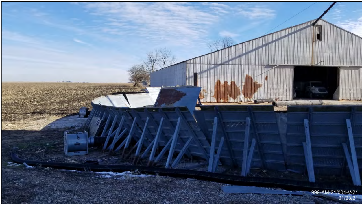
Storage building on Lots 7, 8 and 9, from tracks facing east (proposed grain bin would be past the fencing on this side of the storage building)
