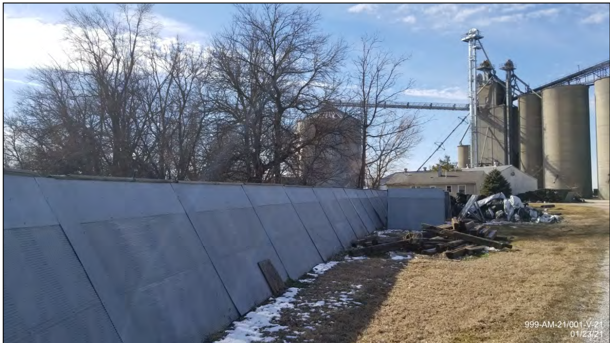
Emergency grain ring section located across street to south of Lots 10, 11 & 12
