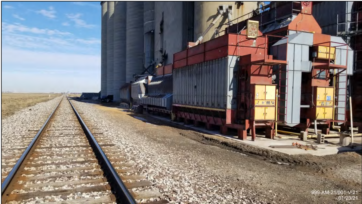
Grain bins along east side of tracks, facing north
