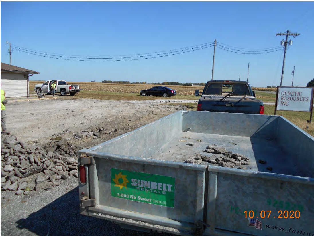
Picture 1505- picture of asphalt in trailer.
