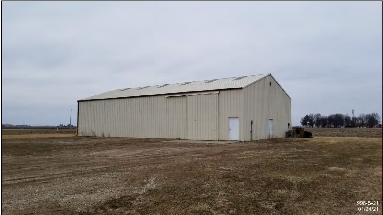
From east side of subject property facing NW to pole shed
