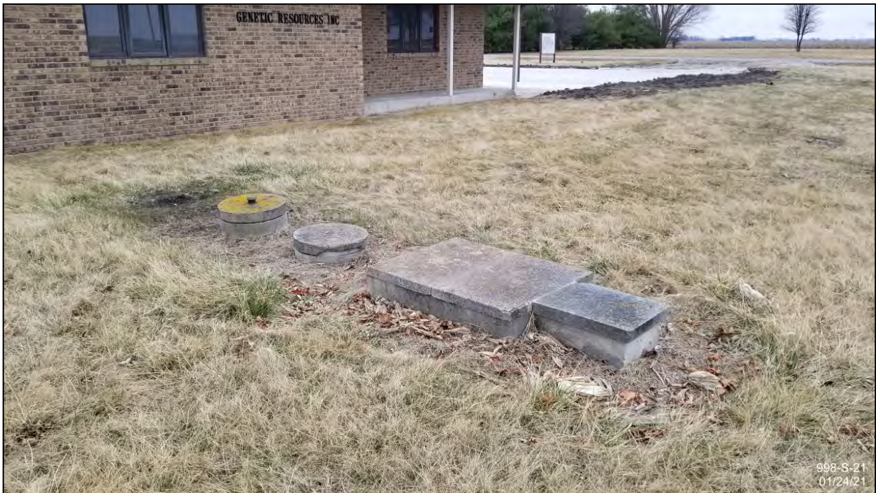
Septic system west of office building
