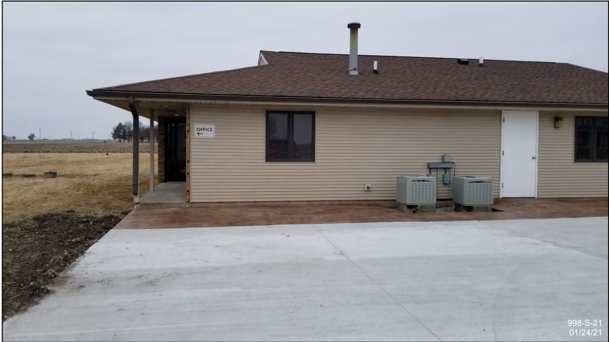
From concrete parking area facing north to office building
