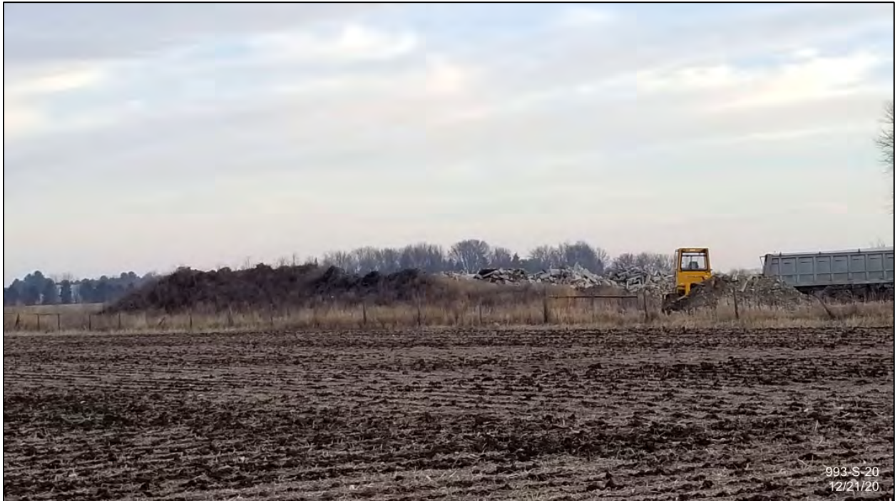
12/2020: from road facing NE toward asphalt millings and demo debris piles
