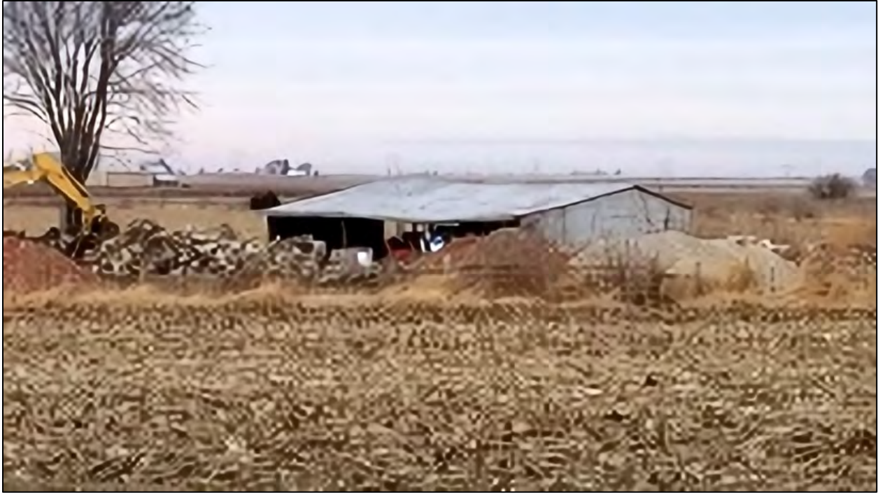
12/2019: From CR 400N facing NW to storage building
