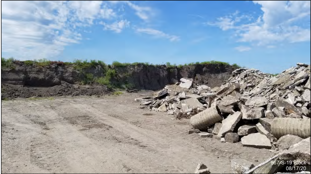
08/2020: from site facing NW toward asphalt millings and demo debris piles
