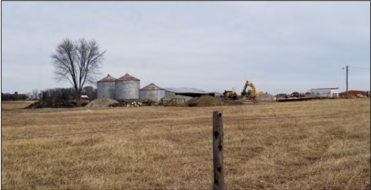
12/2019: from CR 400N just west of 5 acre area facing NE
