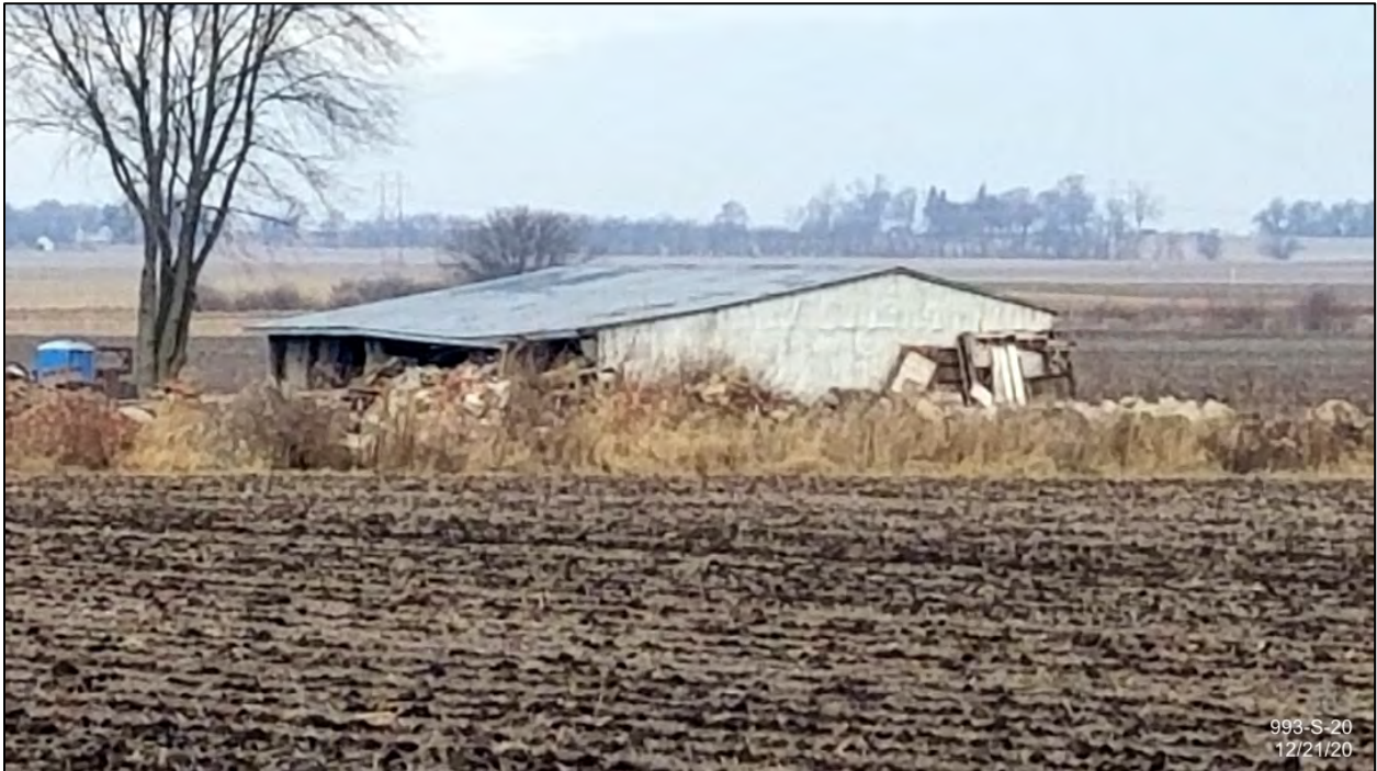
12/2020: From CR 400N facing NW to storage building
