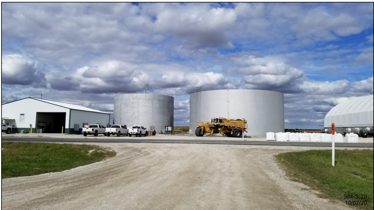
Other buildings in the facility west (left) of hoop building
