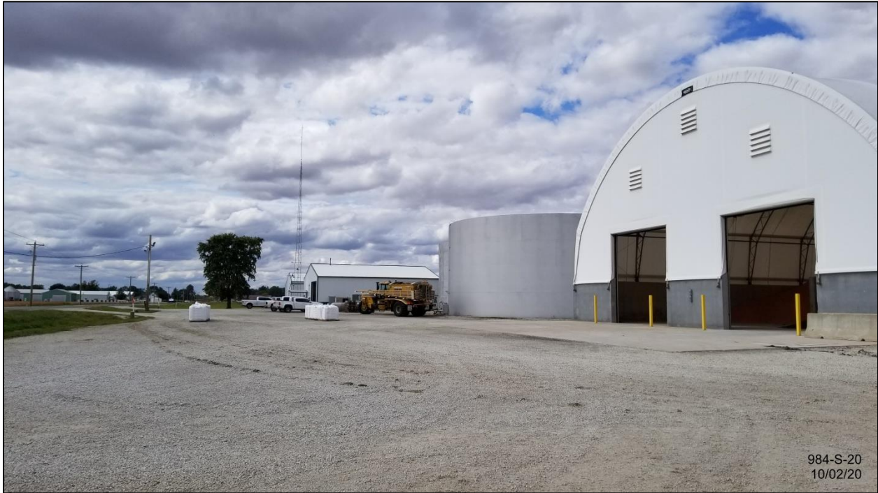
From east end of existing SUP area facing west
