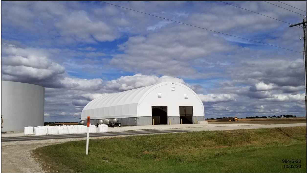
Hoop building in existing Special Use Permit area, from south side of CR 2500N facing NE
