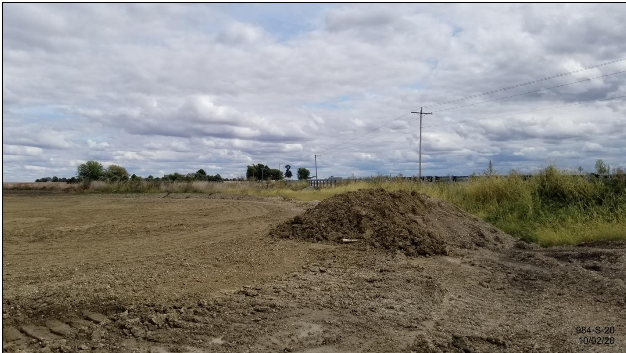
Graded area in proposed SUP area just west of ditch
