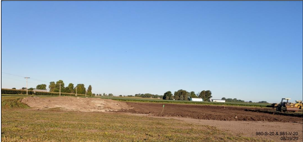
From CR 2000E facing West, close to intersection of CR 2500N
