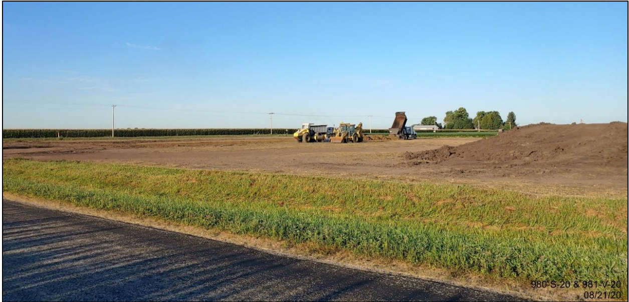
From CR 2000E facing Southwest toward 2500N
