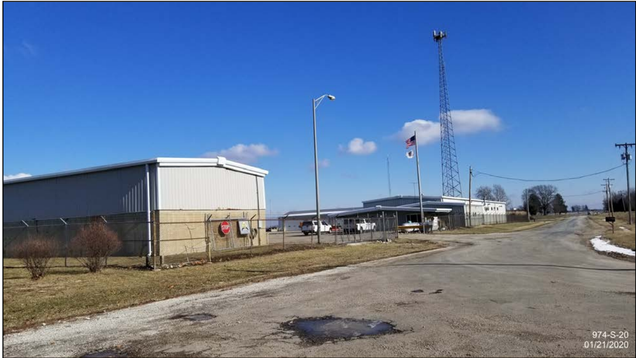
IDOT District 5 Maintenance Facility located northeast of subject property
