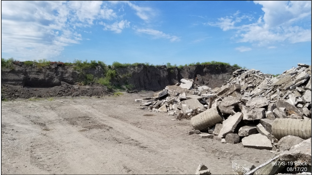
Remaining milled asphalt from Rt 49 project and concrete for crushing in NW corner of 5 acres
