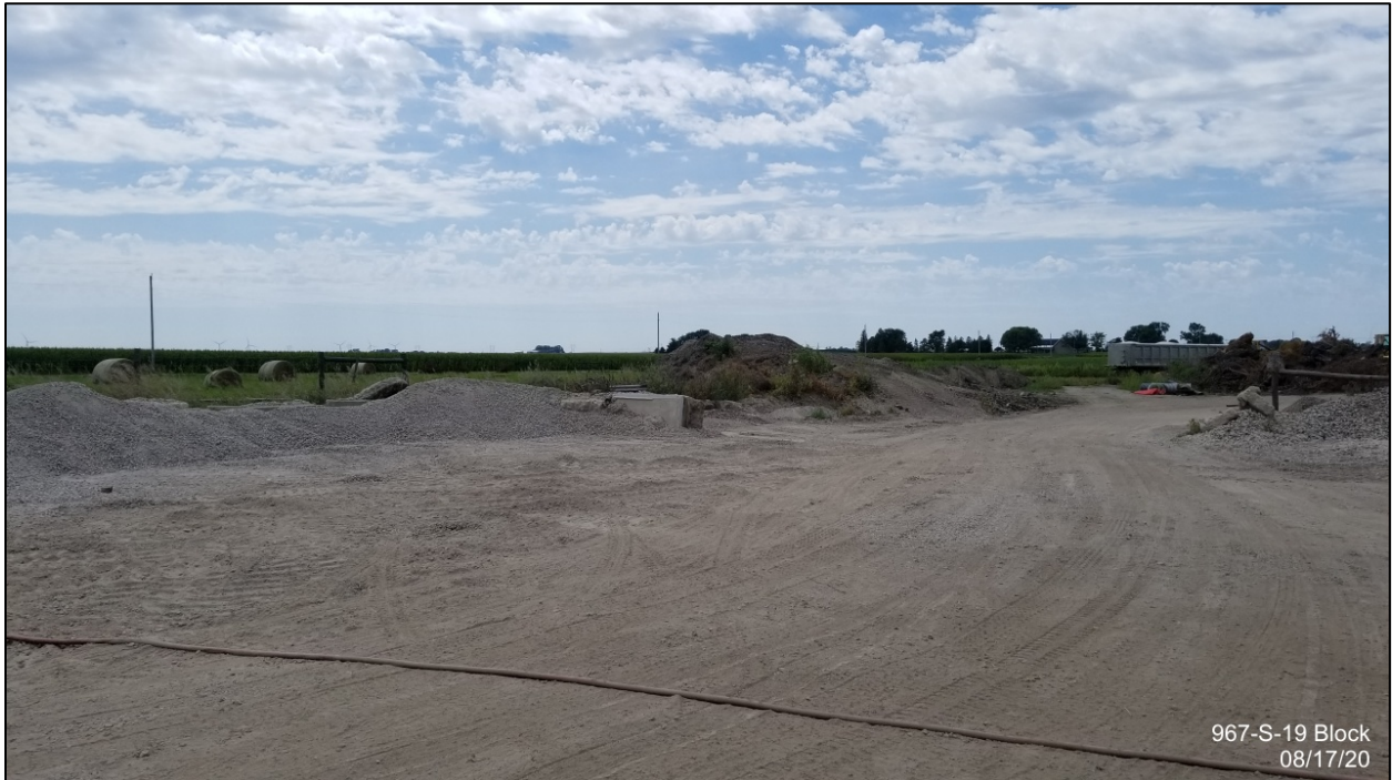
Dirt and crushed concrete stockpiles on west side of 5 acres
