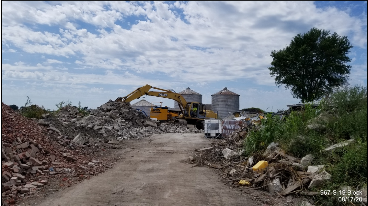
Breaking down concrete for crushing south of existing building
