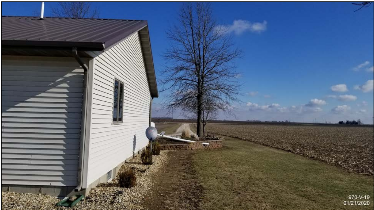
From SW corner of house facing east
