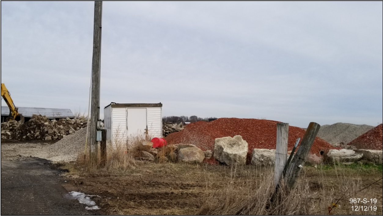
Stockpiles on east side of SUP area
