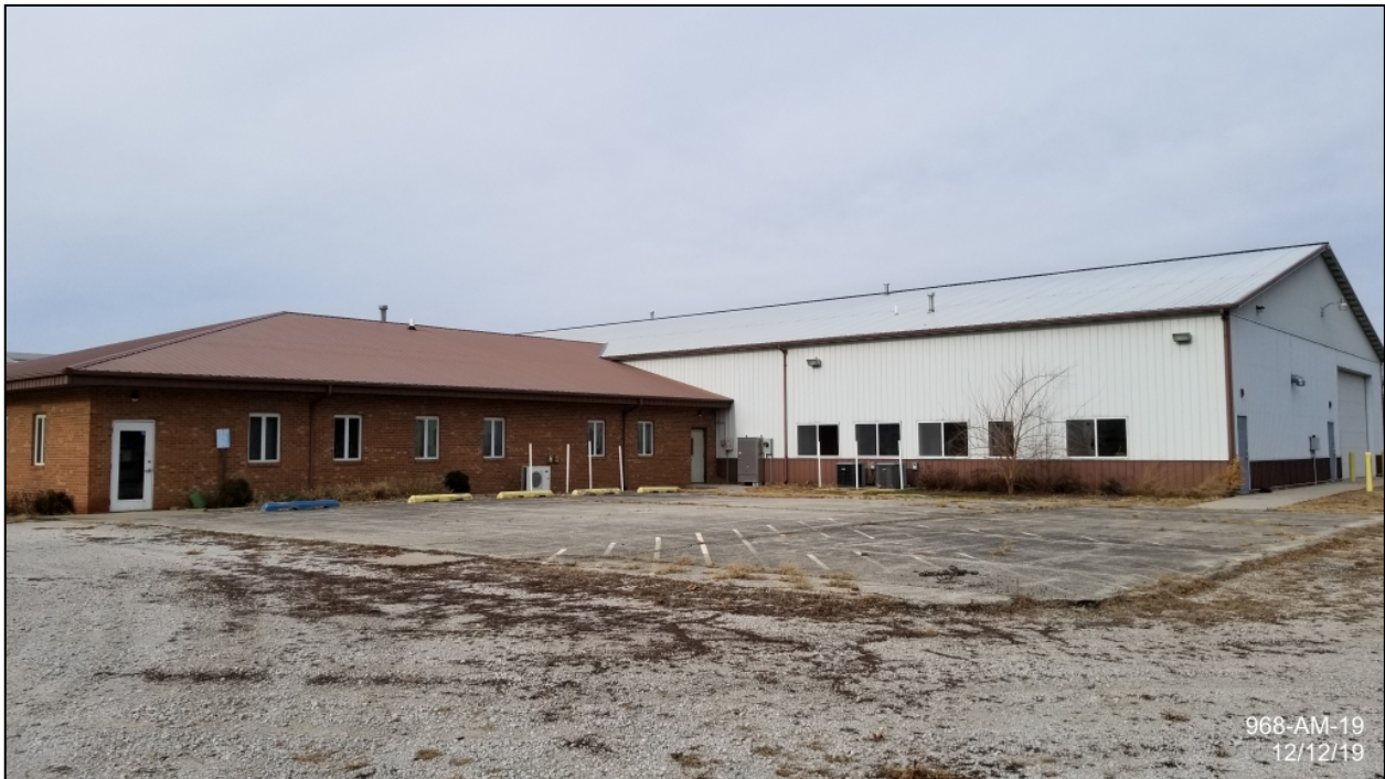
East side of Building 1/Office
