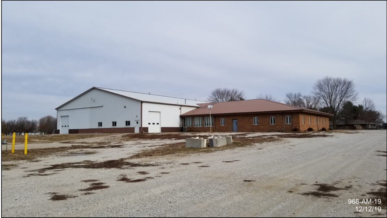
West side of Building 1/Office
