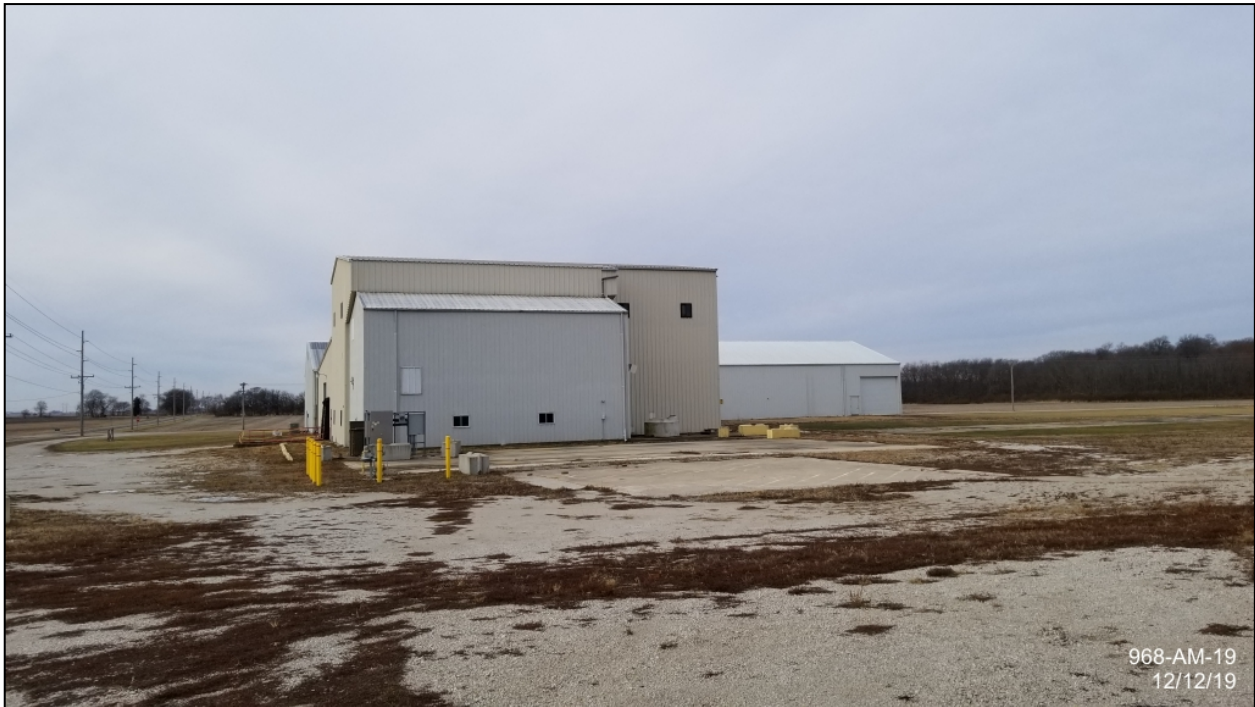
Buildings 2 – 6 taken from Building 1 facing west
