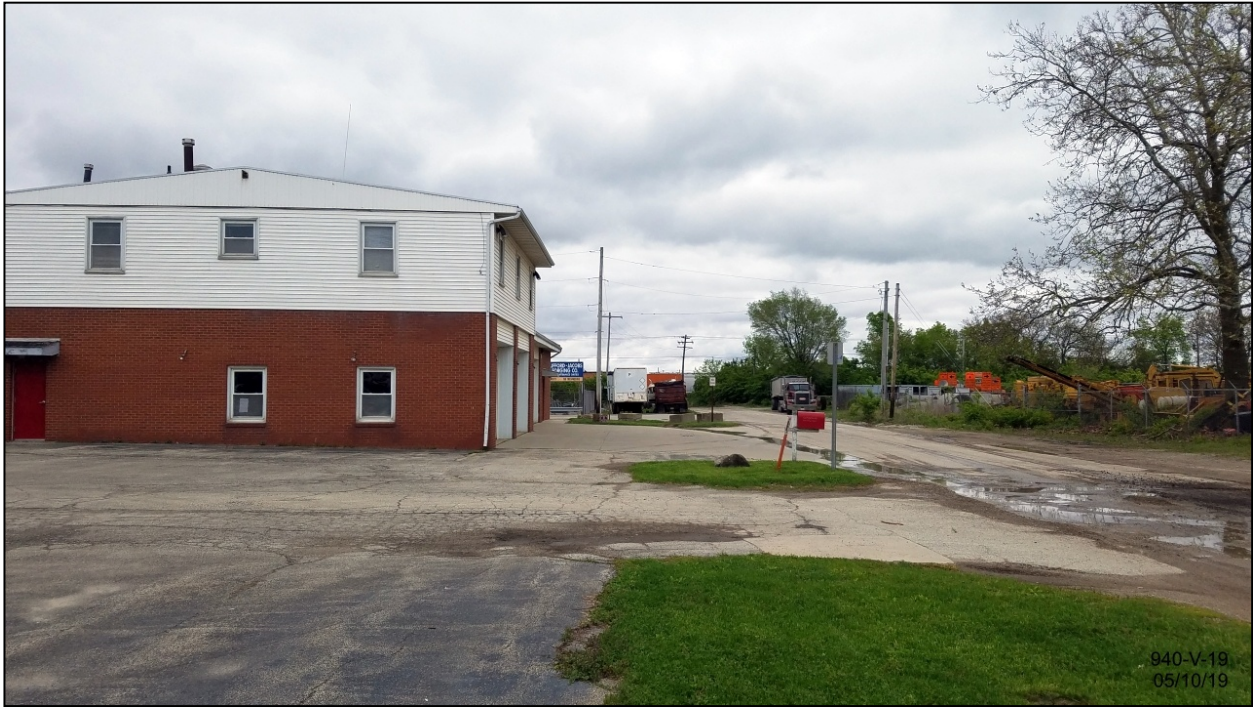
From west edge of parking lot, facing east
