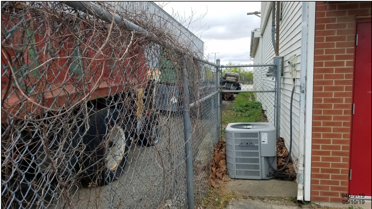
From fire station parking lot, facing east
