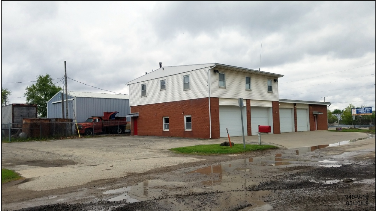
Fire Station, from Wilber Avenue facing NE
