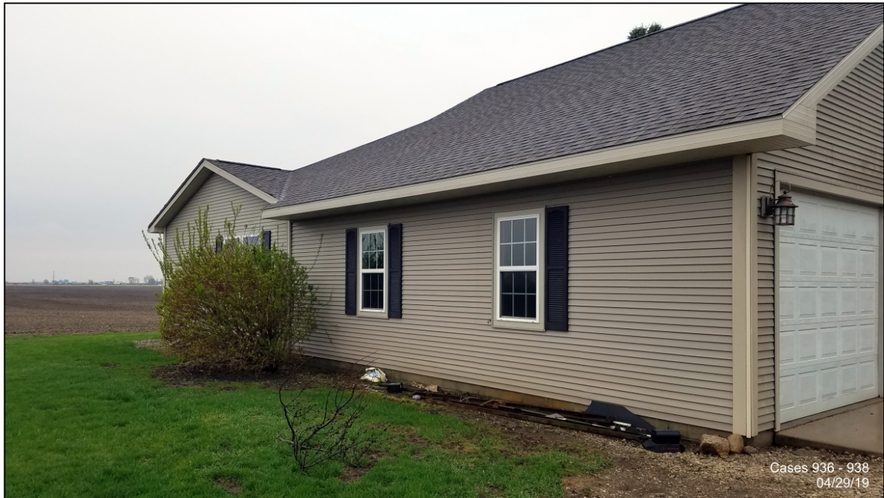
North side yard, facing southeast
