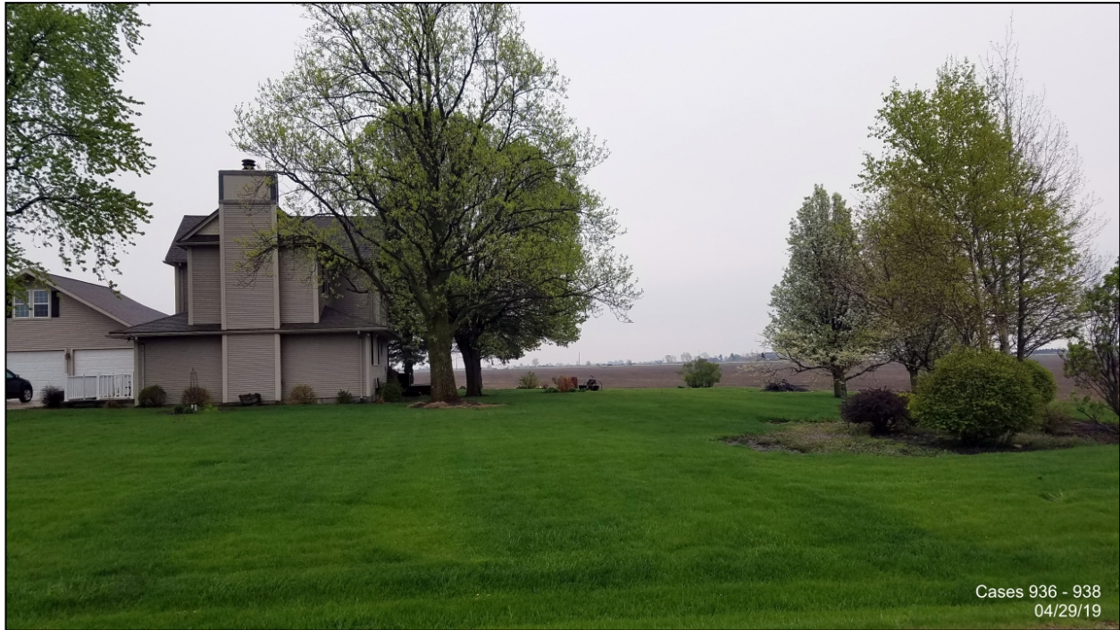
From CR 1400E facing east
