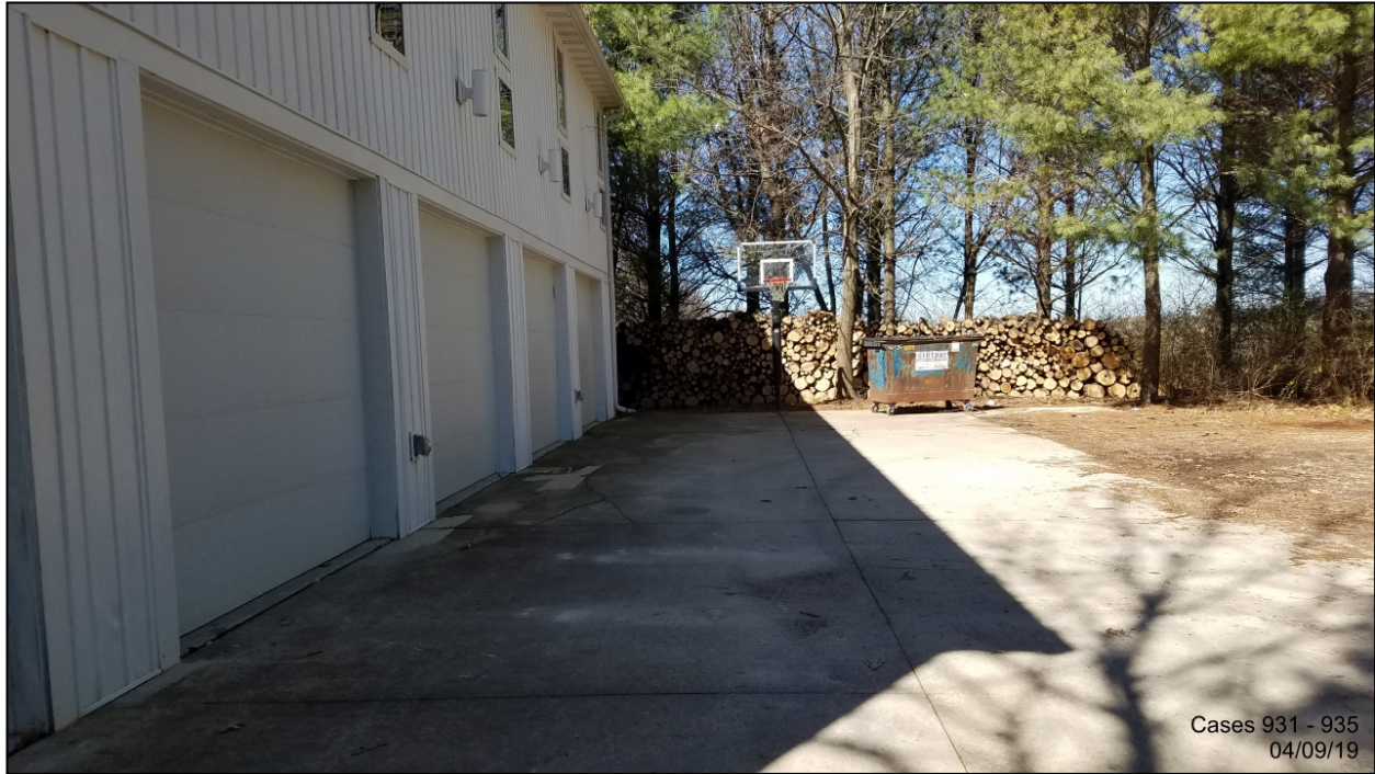
Detached garage with residence on 2 nd floor, on proposed lot 3 Concrete pad is area for accessible parking for events
