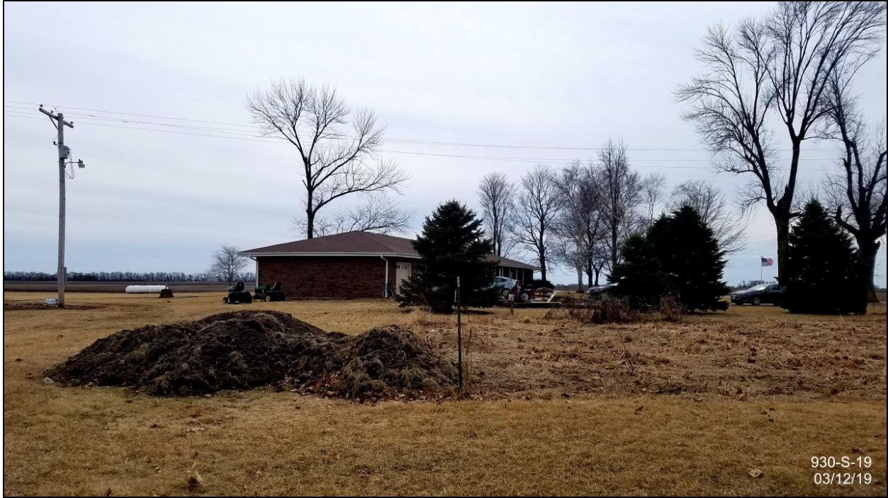
From access drive north of property facing south to residence
