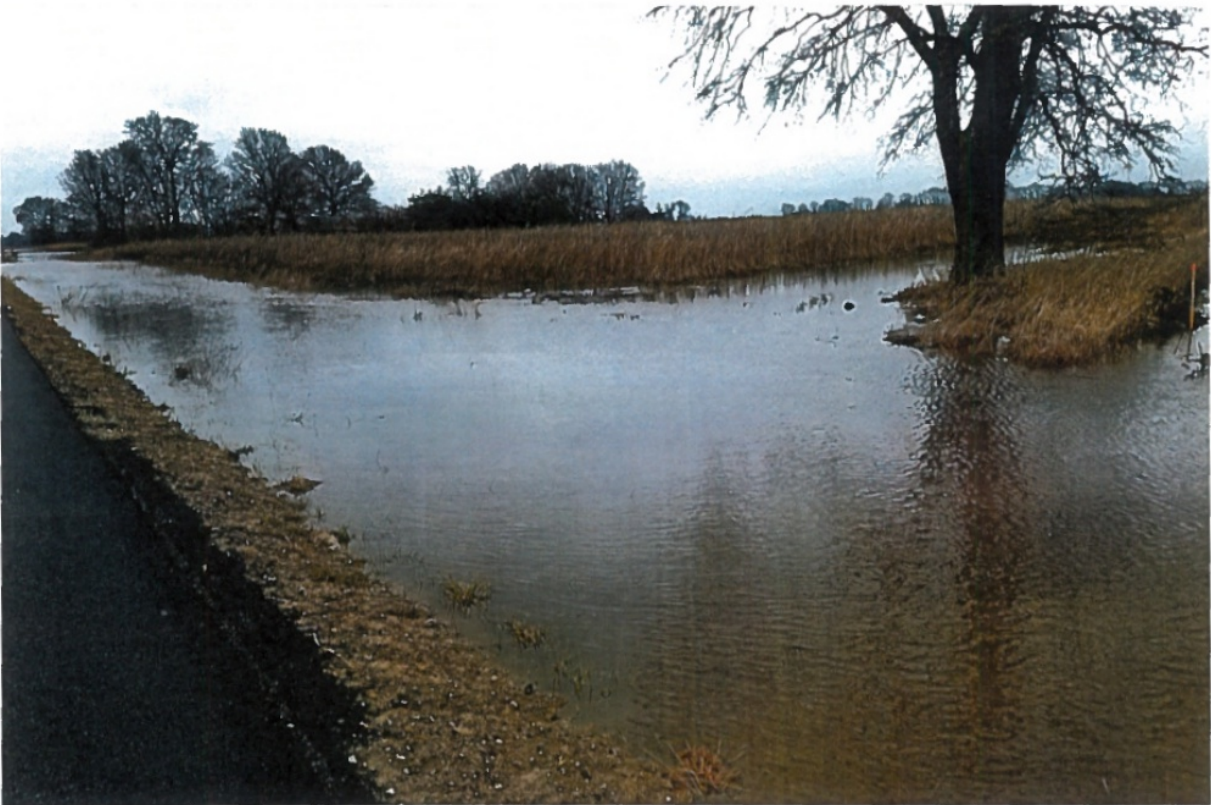
US 45 roadside ditch at southwest corner of subject property
