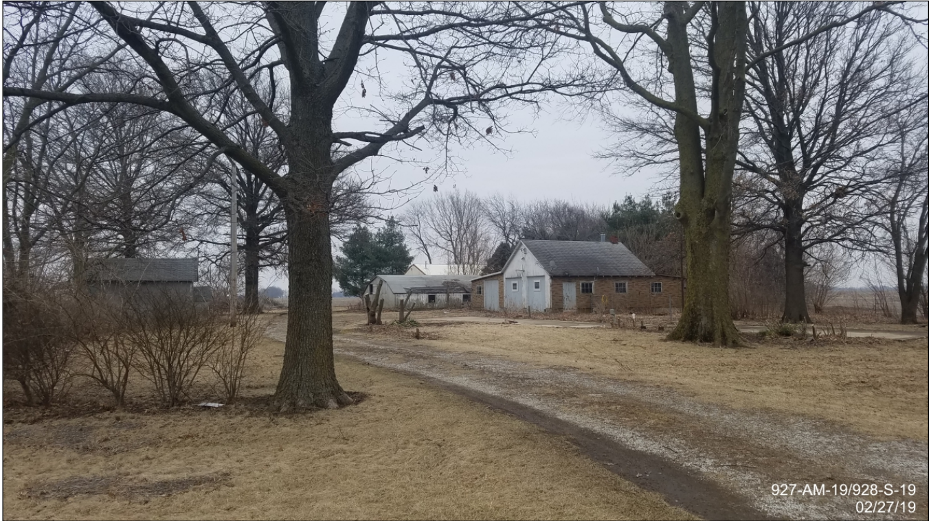
From US 45 facing east
