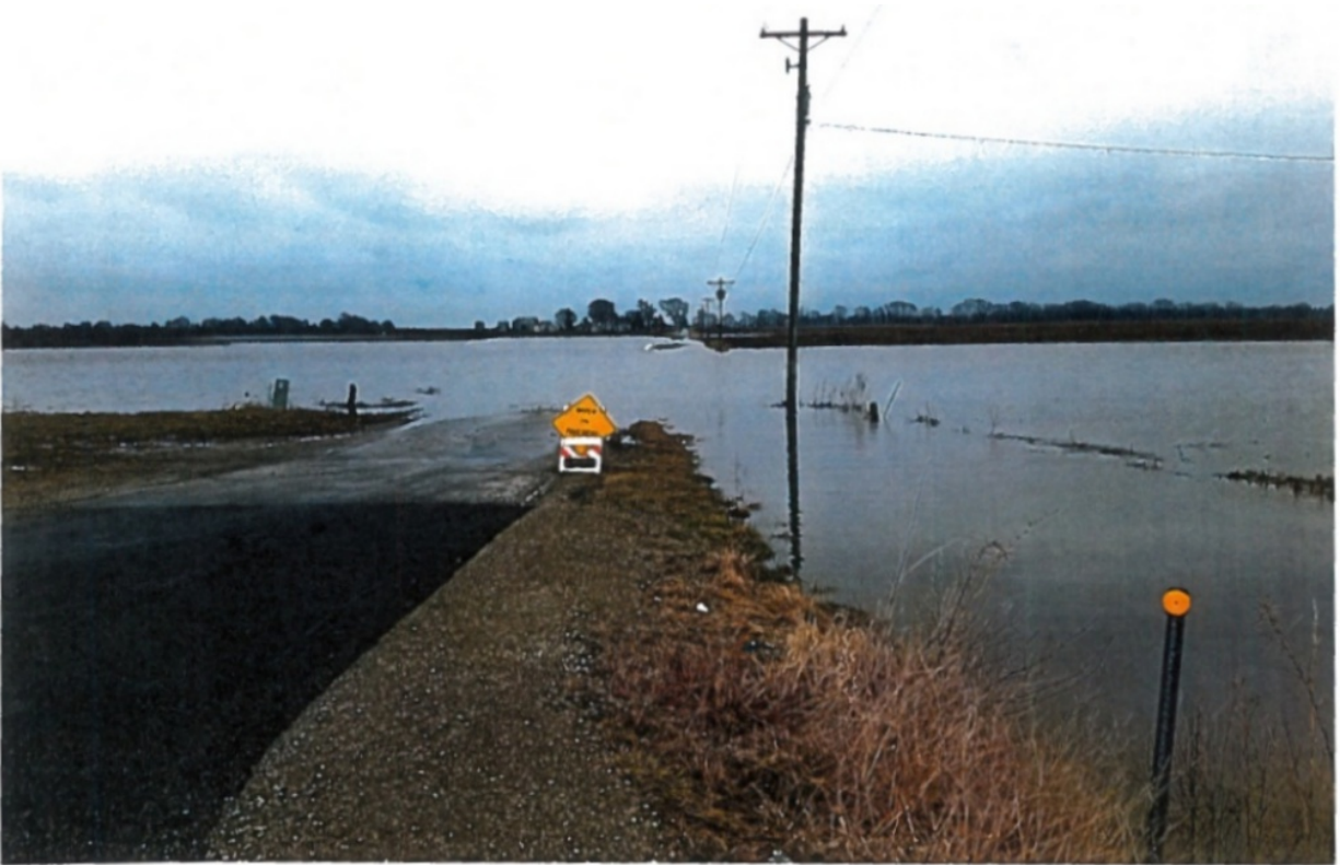
At SE corner of Olympian at US 45 facing east, subject property is at right
