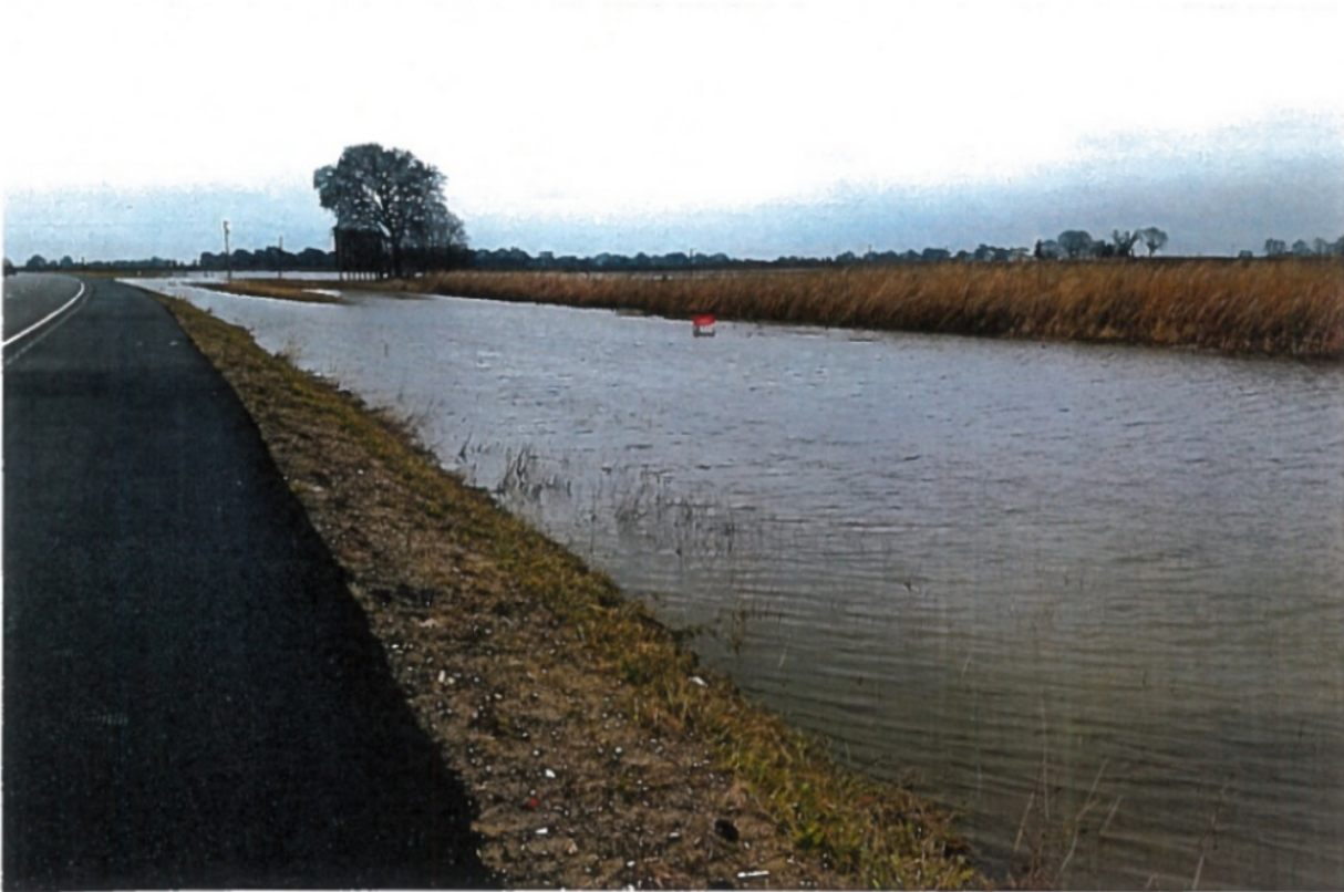
US45 roadside ditch north of existing structures facing northeast
