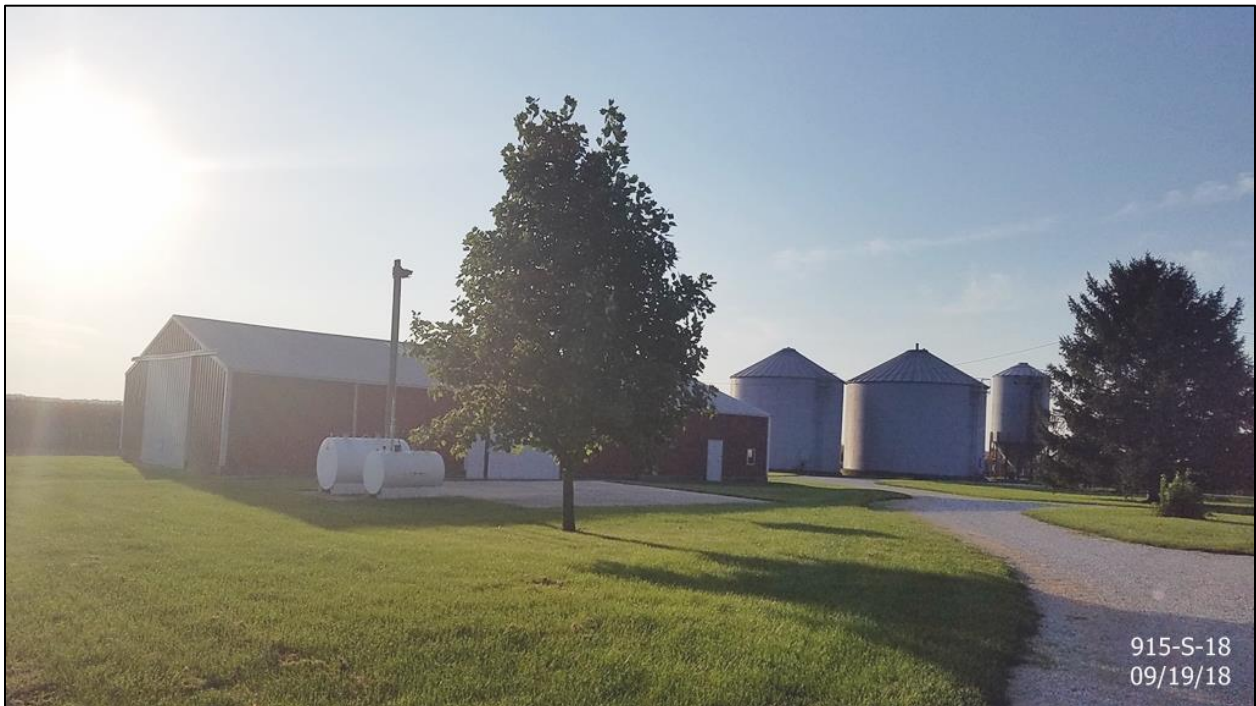
Existing accessory buildings, from driveway facing southeast
