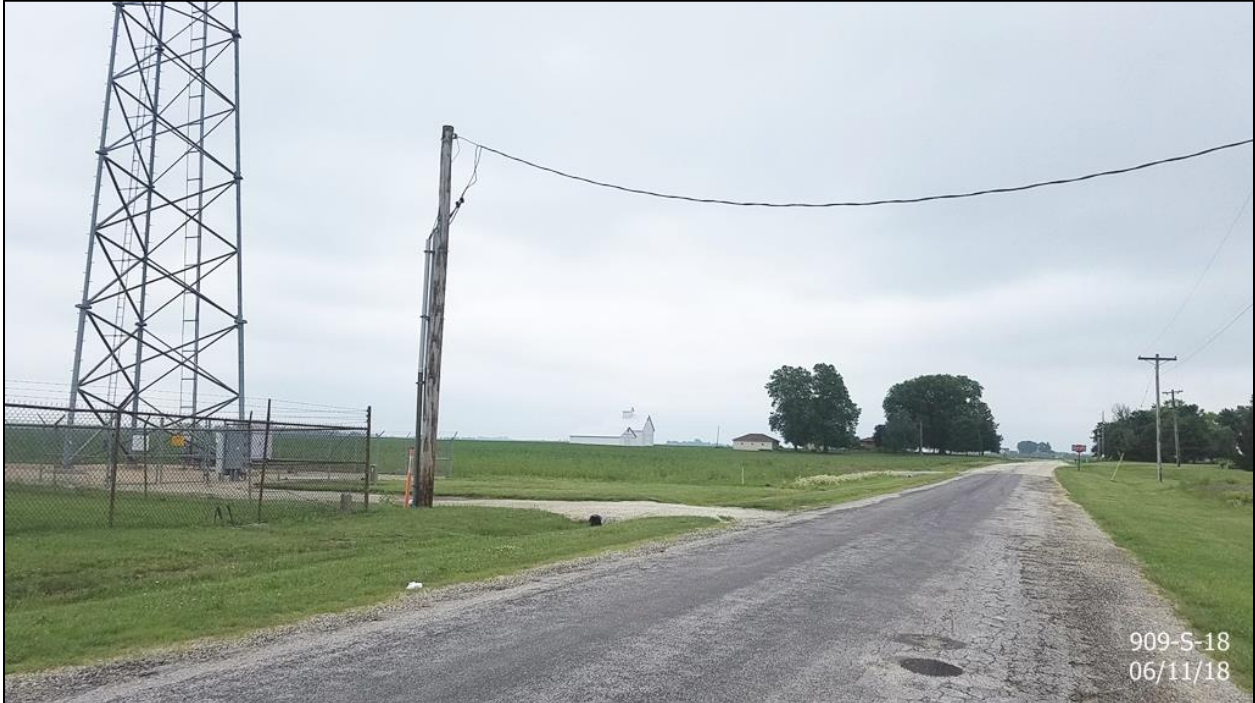
From Leverett Rd (west of curve) facing east – subject property is on left side of road past the cell tower
