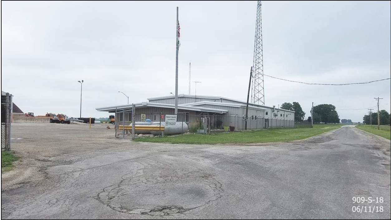
From Leverett Road west of IDOT storage facility, facing ENE
