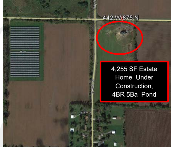
Portage Solar Farm (Solar Farm 2) October 2016
