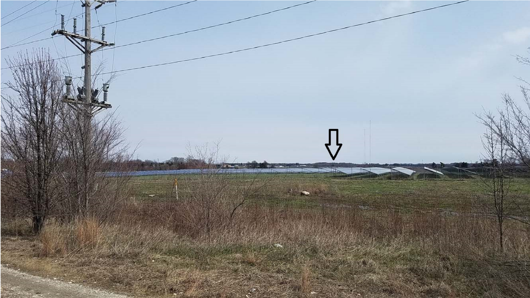
UIUC Solar Farm distance: ~250 feet to closest panel (arrow) taken from railroad tracks 04/05/18
