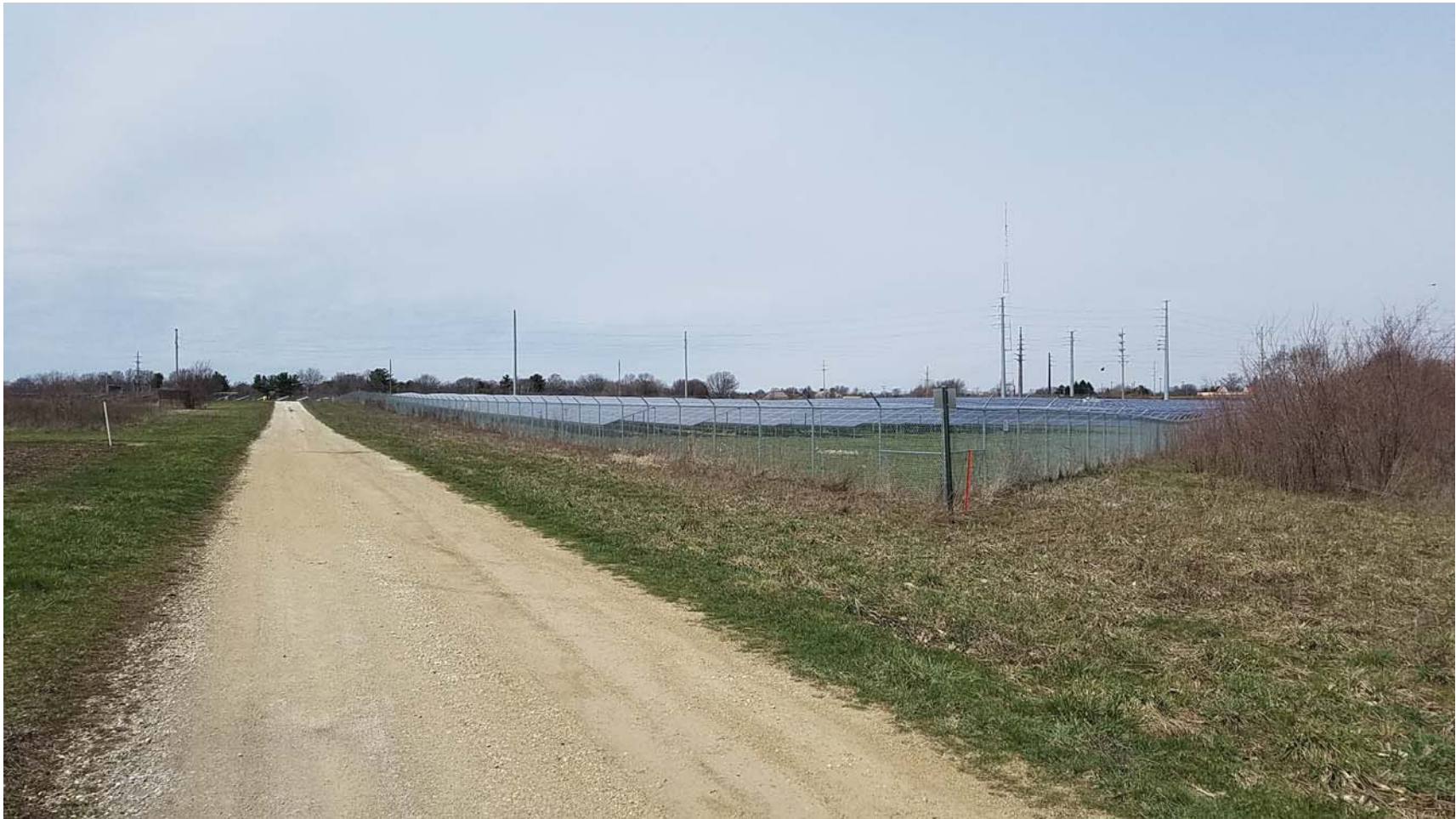
UIUC Solar Farm distance: ~200 feet to closest panel 04/05/18
