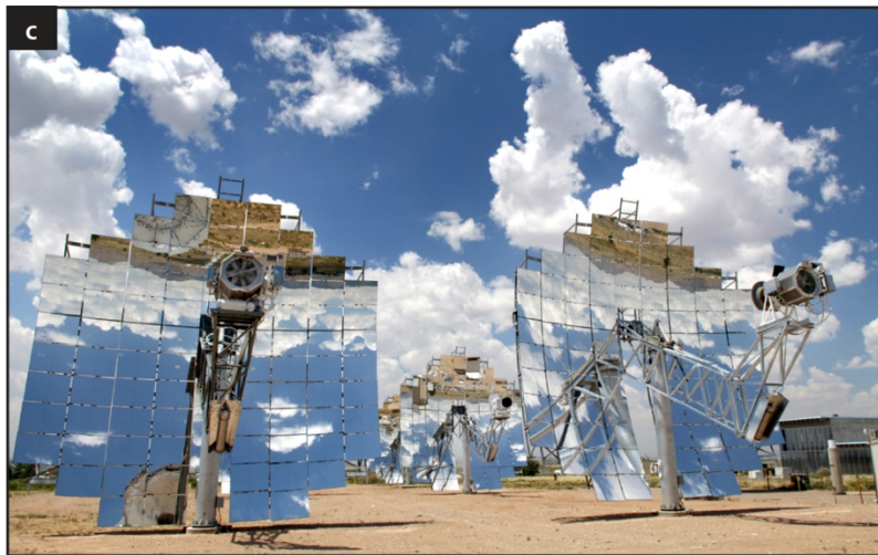
FIGURE 1-1 Typical Solar Fields for Various Technology Types: (a) Solar Parabolic Trough (Source: Hosoya et al. 2008), (b) Solar Power Tower (Credit: Sandia National Laboratories. Source: NREL 2010), (c) Dish Engine (Credit: R. Montoya. Source: Sandia National Laboratories 2008), and (d) PV (Credit: Arizona Public Service. Source: NREL 2010)
