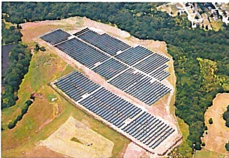
Figure 1: Utility-scale solar facility (5 MW AC ) located in Catawba County. Source: Strata Solar
