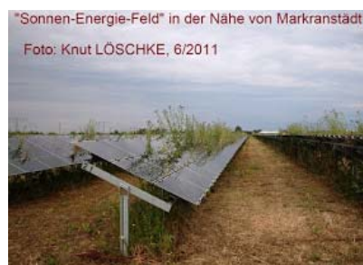
photo by Knut Loschke This a photo of a Solar Farm near Markranstädt,
