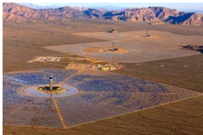
Ivanpah Solar Electric Generating System Image via http://www.energy.ca.gov
