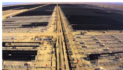
Image: BHE Renewables Topaz Solar Farms construction site, Carrisa Plains, CA
