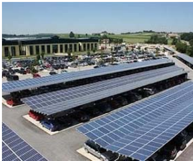
Photo: Clean Technica Solar carports have a double benefit: generating renewable energy and reducing the island heat effect
