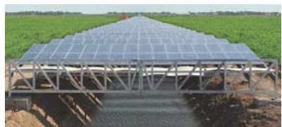
Narmada Canal solar power project in India saves agricultural fields for farming
