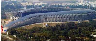
Dragon-Shaped Solar Stadium in Taiwan is 100% Powered by the Sun Read more: Dragon-Shaped Solar Stadium in Taiwan is 100% Powered by the Sun
