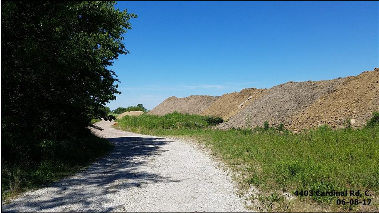
SE corner of subject property facing west – material stockpiles
