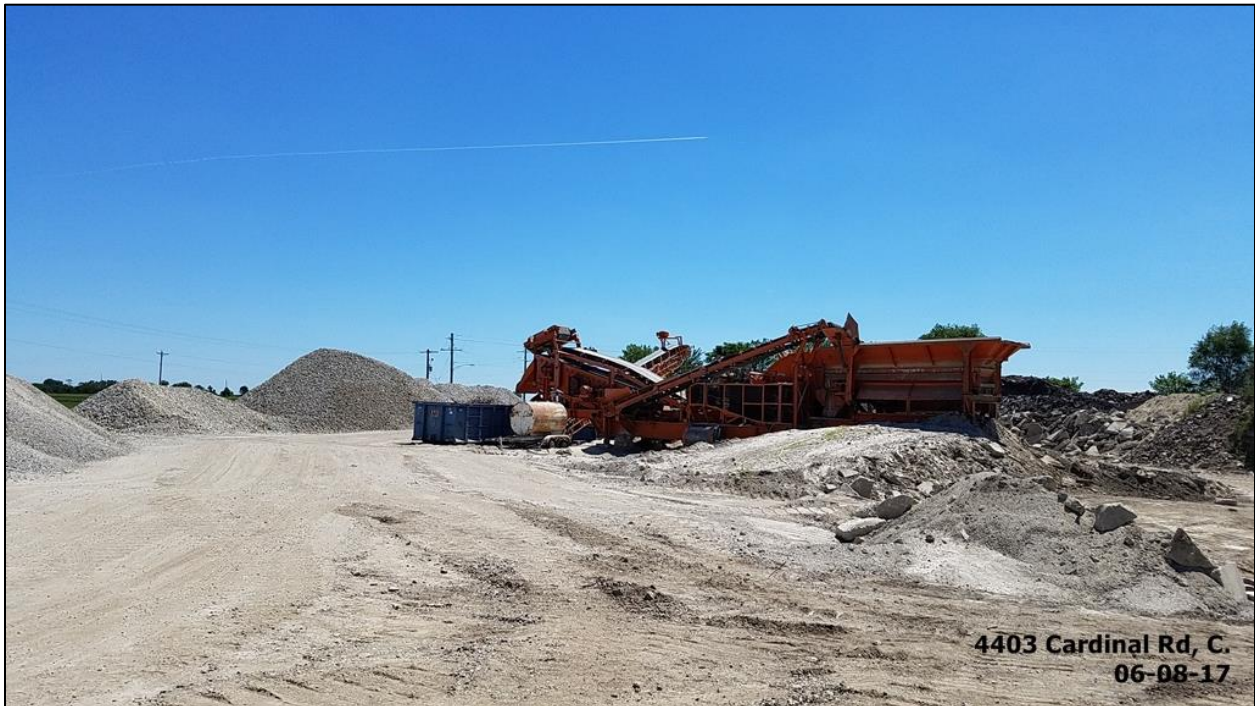
NE corner of subject property - material stockpiles and concrete crusher
