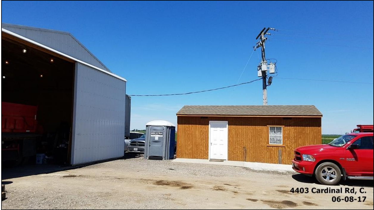
NW corner of subject property – shed and office (no permits on file)
