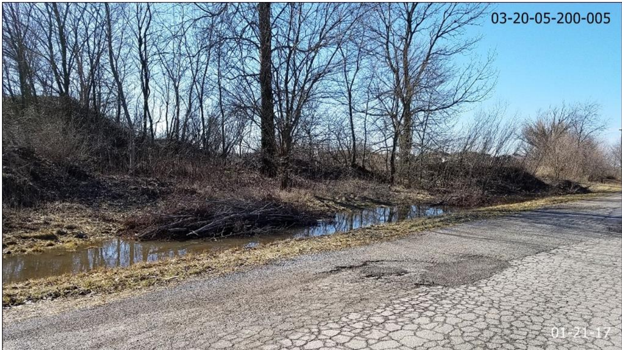
Yard waste blocking drainage ditch along Cardinal Rd west of Staley Rd
