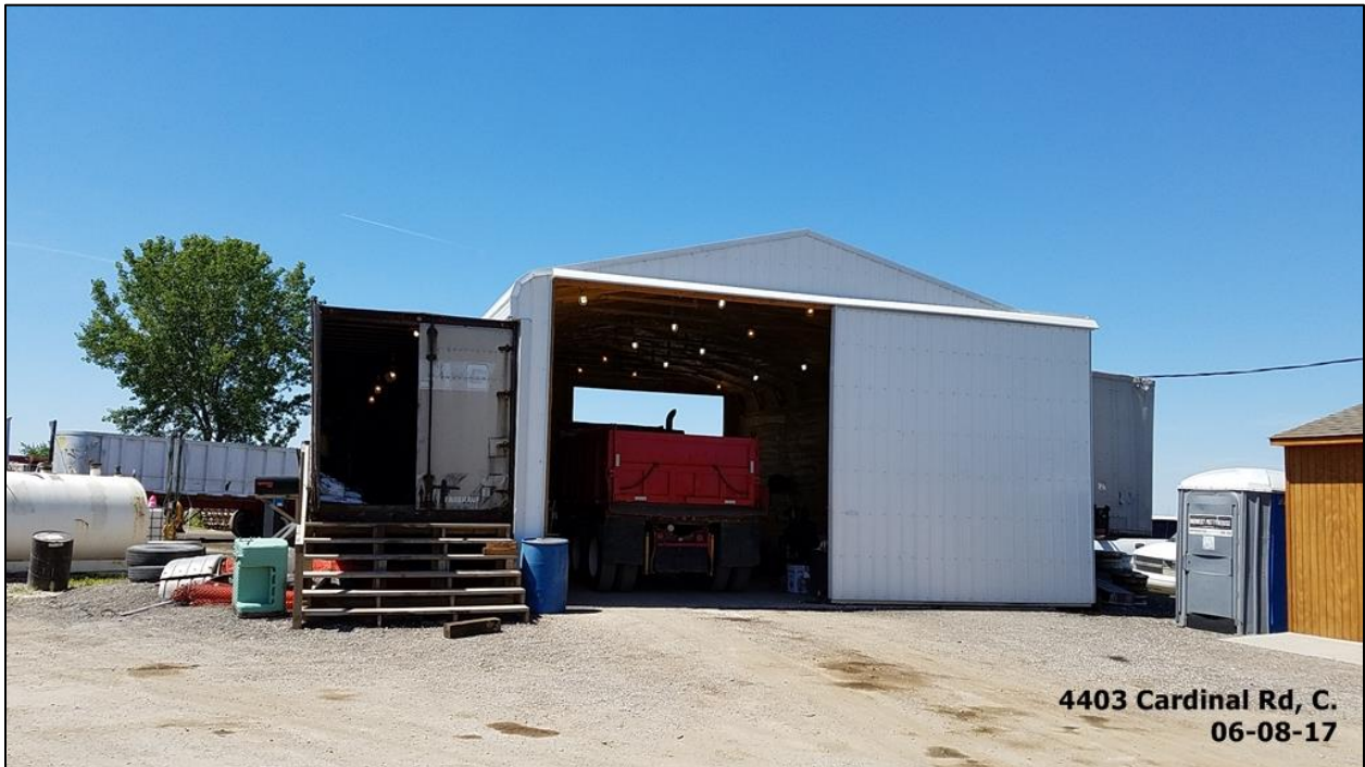
NW corner of subject property – shed with semi used as storage
