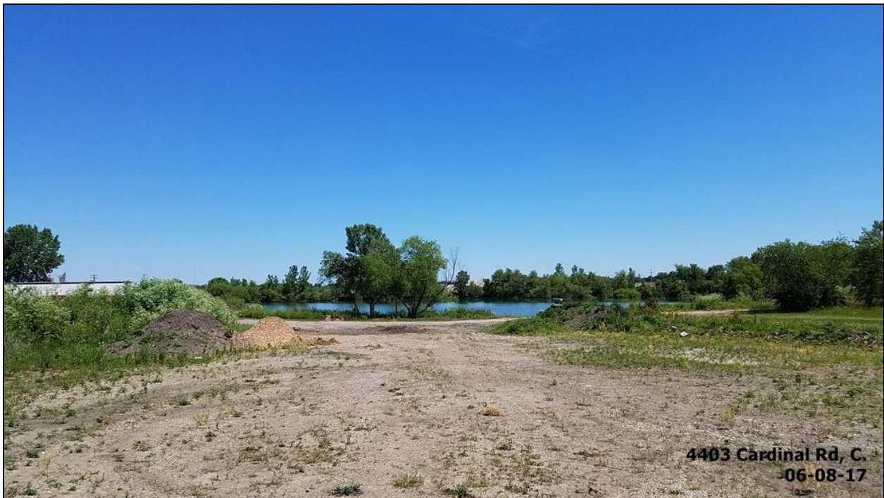
SW corner of subject property facing NW – material stockpile area (only small stockpiles)
