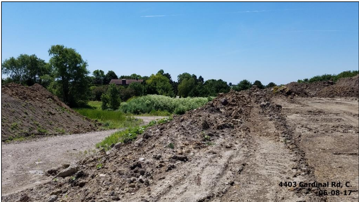
SE corner of subject property – material stockpiles
