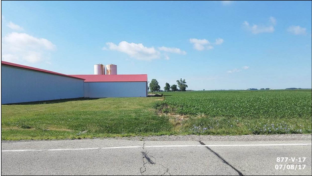
West side yard, facing south from US 136
