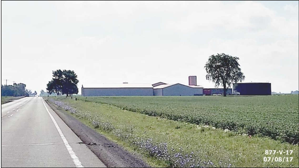
Subject property from US 136 facing east
