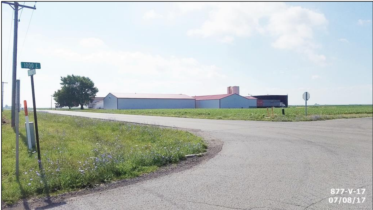
Subject property from intersection of US 136 and CR 1000E, facing southeast
