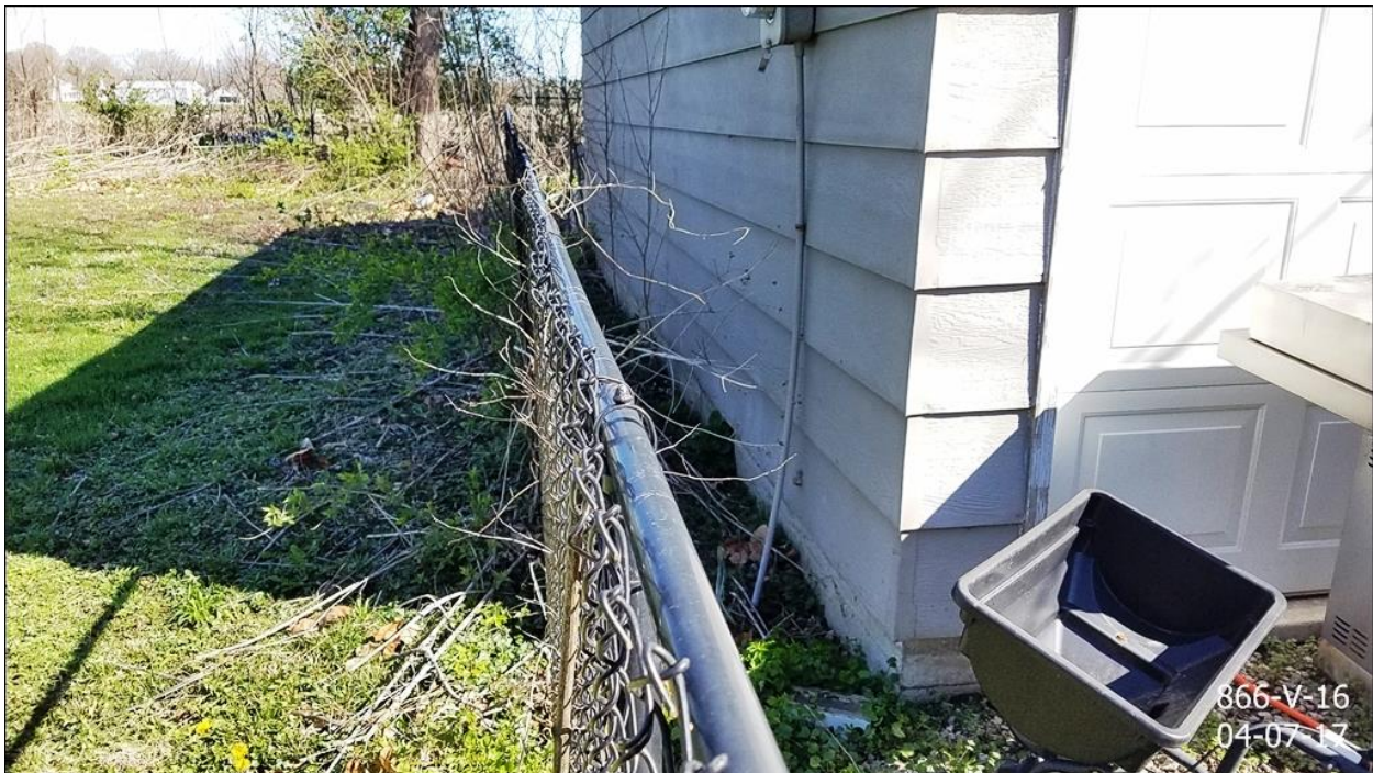
Shed side yard, facing north
