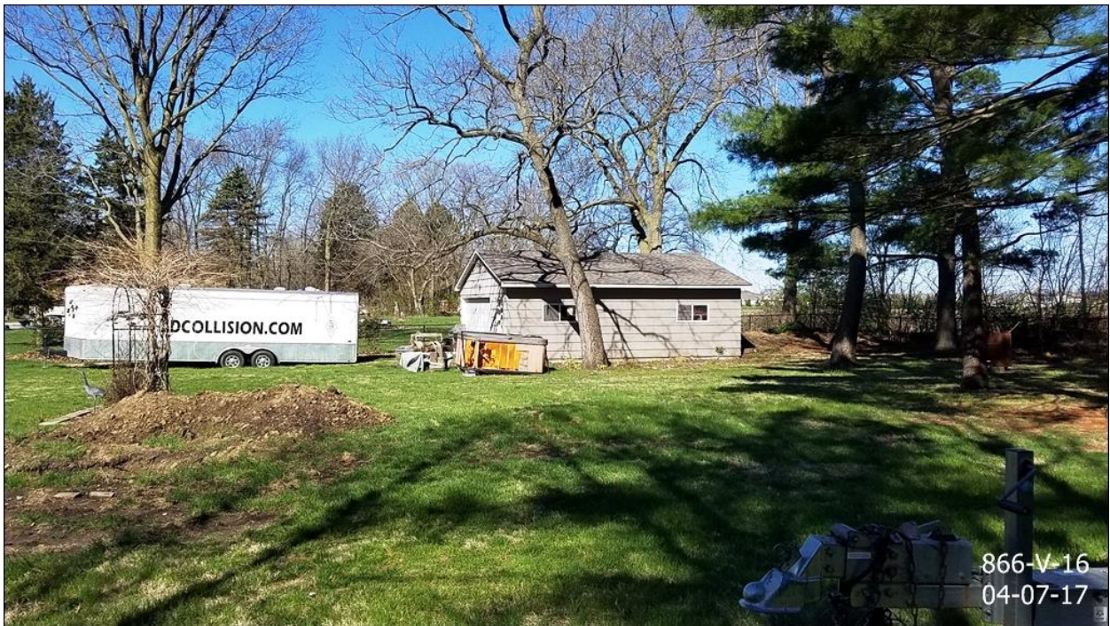
Subject shed, taken from east side of back yard, facing west
