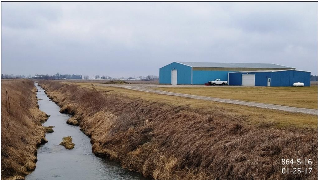
From Kaskaskia Ditch bridge on Bradley Avenue facing southwest
