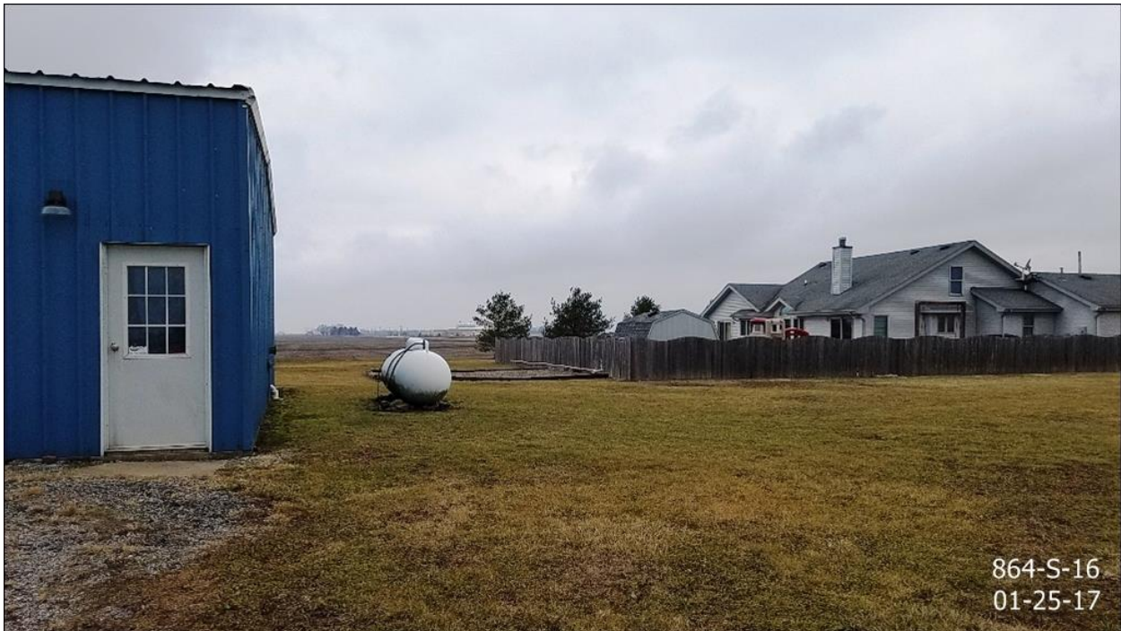
From east side of smaller part of barn, facing west
