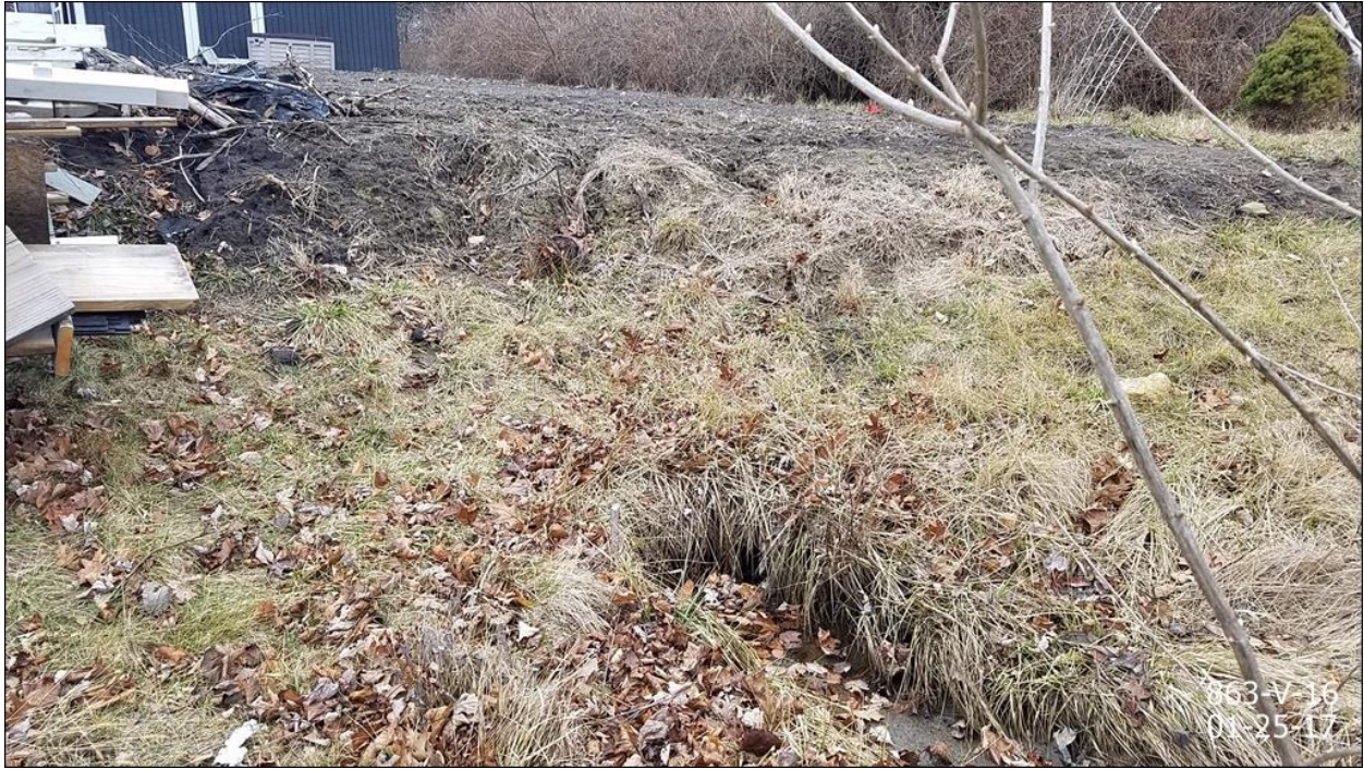
Drainage outlet on southeast corner of subject property, drains to...
