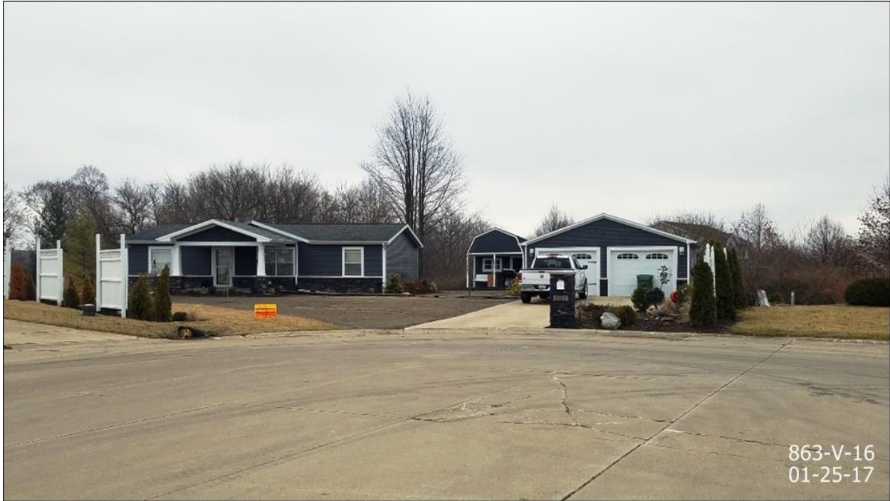
Subject property from west, facing east-northeast
