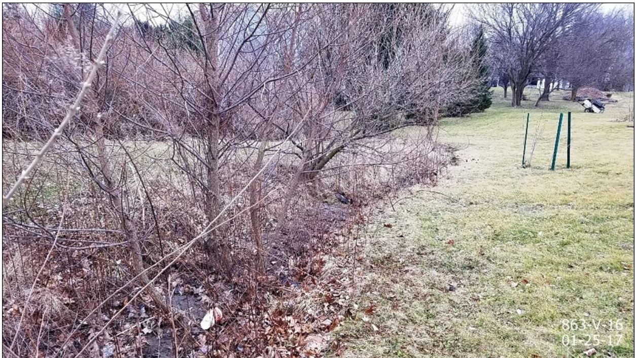
Drainage ditch extending from subject property through property to the south
