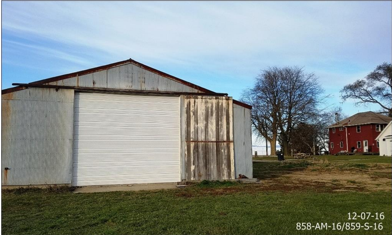
Barn for proposed Events Center from south side; petitioner's residence and accessory shed on right
