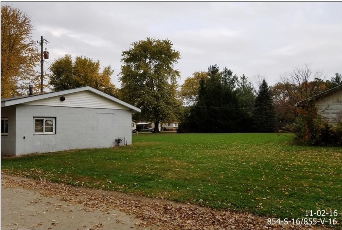
Former MHP Management Office (sits too close to property line)
