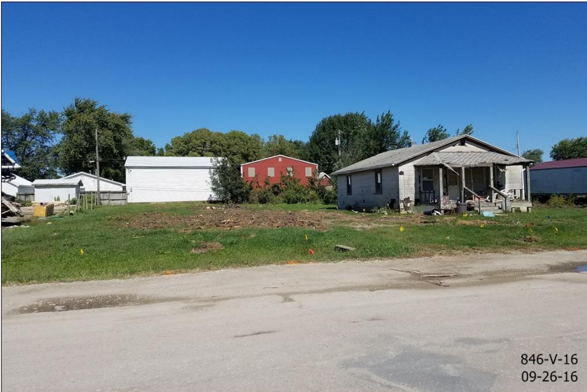
Recently demolished residence where addition will be constructed
