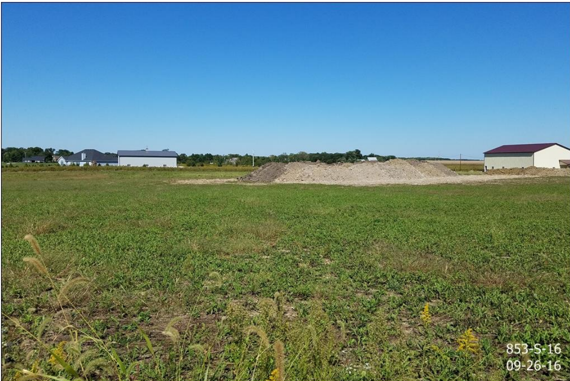
Pond stockpiles near neighbor's building, from CR 500E facing northwest
