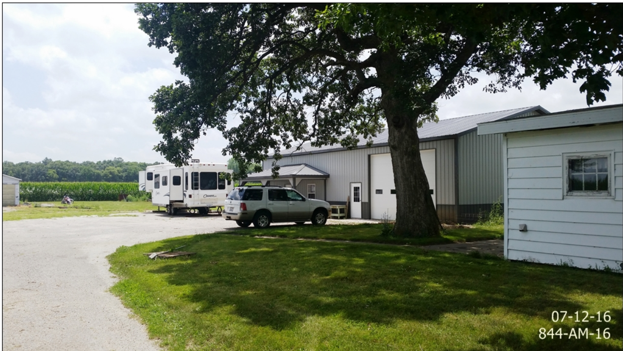
Machine shed (former restaurant)
